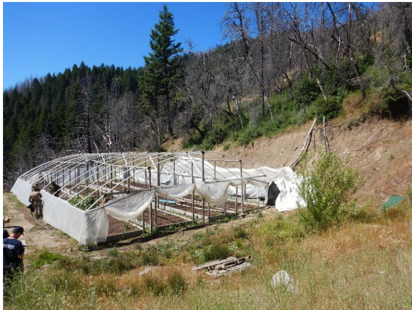
photo 12—Looking south at graded flat cut into hillslope at WQ 10. Note concentrated vegetation between greenhouse and photographer where water is emanating from the subsurface.
