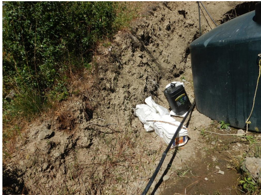
photo 10 —Looking south from top of the reservoir's impounding buttress in the vicinity of WQ 9.
