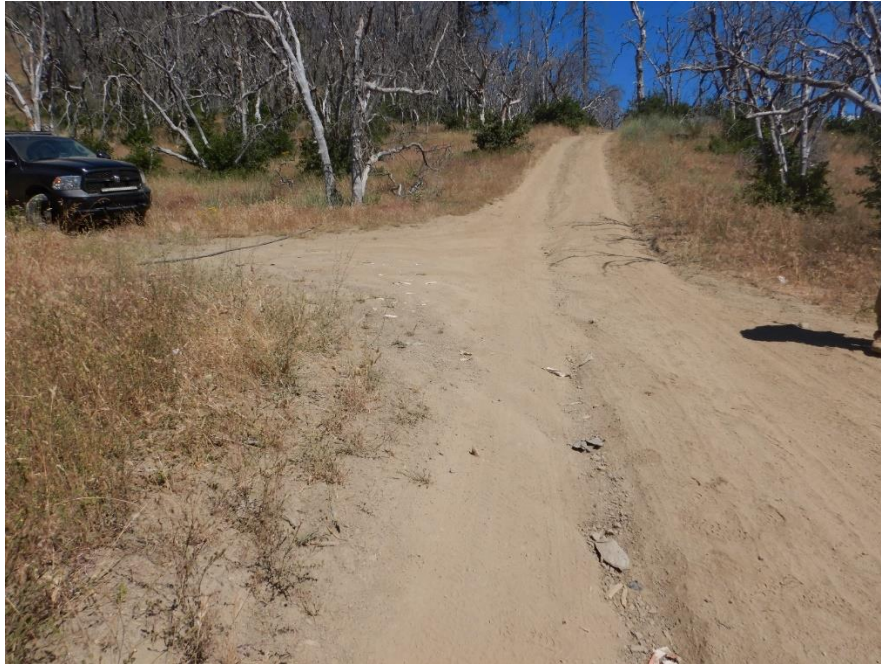
photo 5 —Looking north up steep, unarmored road with ruts and loose, fine sediment.
