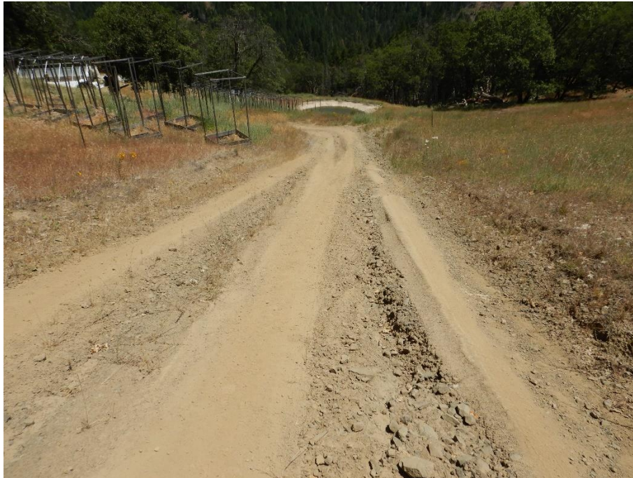
Photo 1—Looking northeast towards the Mad River from WQ 1. Note steep road with a surface of fine sediment and ruts.
