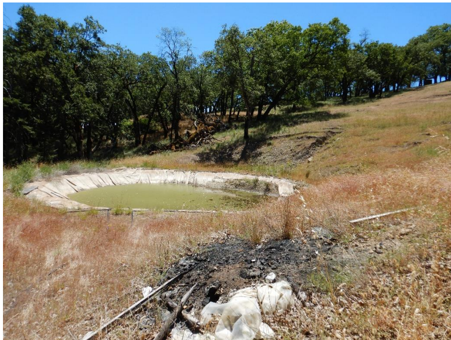
Photo 2—Looking at pond located at WQ 2. Note sediment covering pond liner on upslope side.
