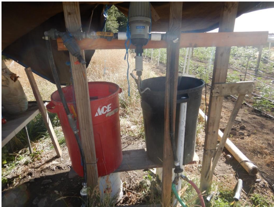
Photo 12—Fertilizer mixing tanks located at WQ 7.
