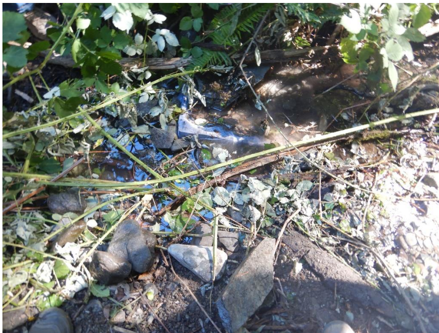
Photo 9—Lid to box can be seen in the middle of the image. The box was placed in an excavated hole in the stream bed to facilitate the diversion at WQ 4.
