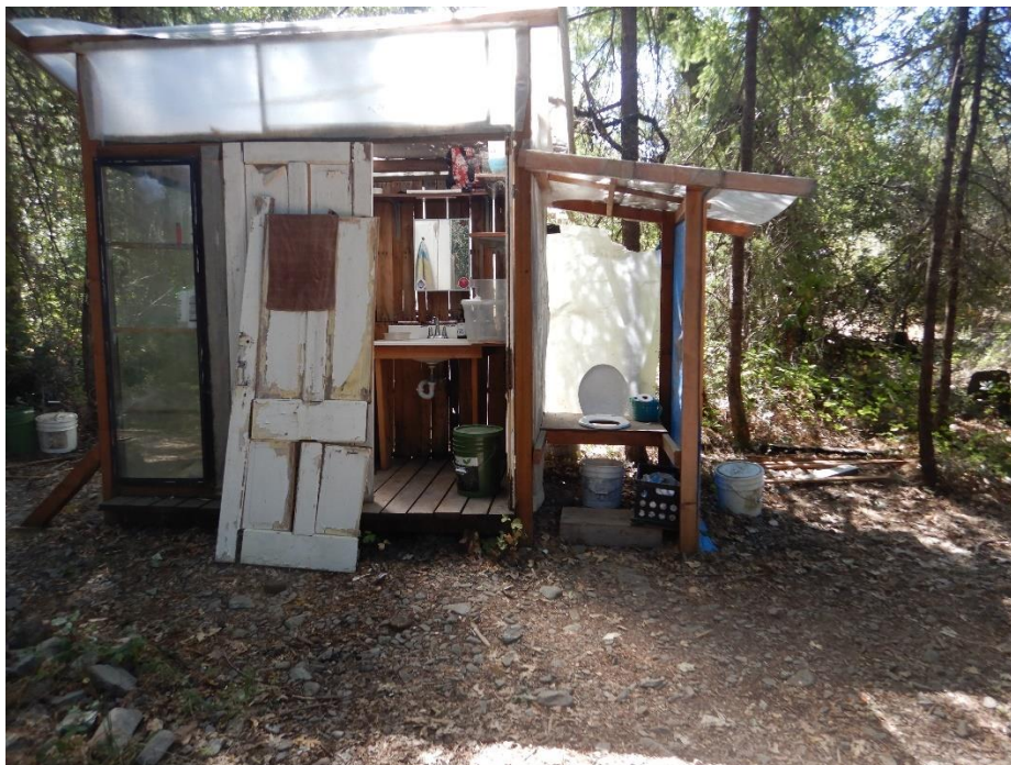
Photo 18—Toilet and shower at WQ 10. Human waste is collected in a bucket.
