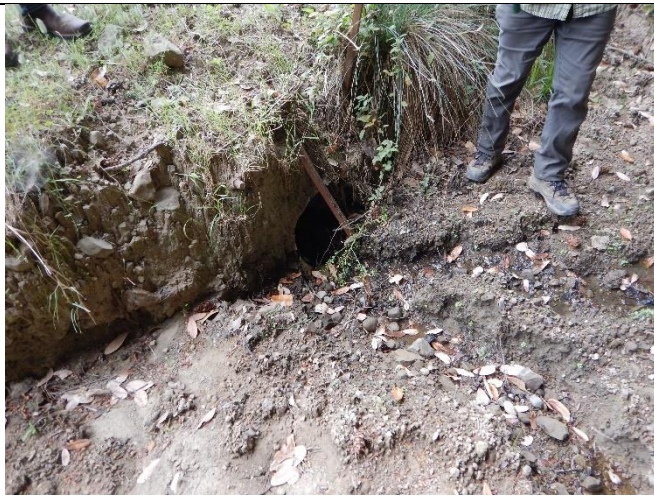
Photo 5 – FR2; perched outlet of culvert with sediment placed above the culvert from roadwork
