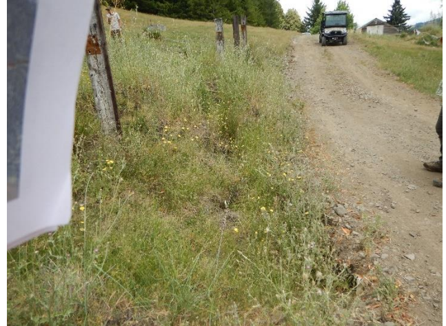
Photo 18 – FR13; ditch relief culvert
