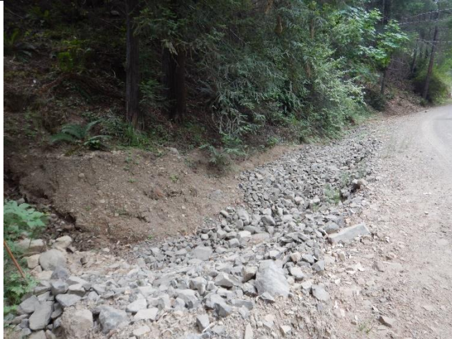
Photo 1 – FR1; inboard ditch and stream entering culvert
