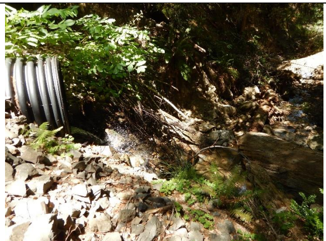
Photo 24 – FR18; perched outlet of culvert stream crossing
