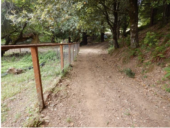
Photo 17 – FR12; stretch of insloped road with inboard ditch discharging to stream crossings FR10 and FR11
