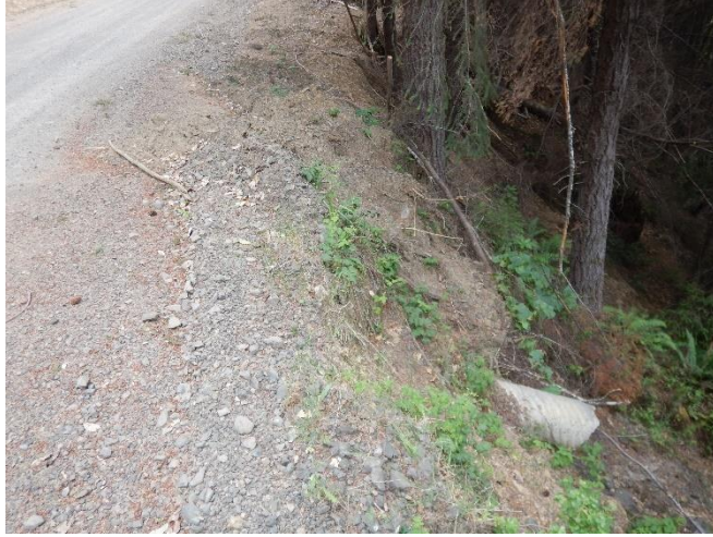
Photo 5 – FR2; perched outlet of culvert with sediment placed above the culvert from roadwork
