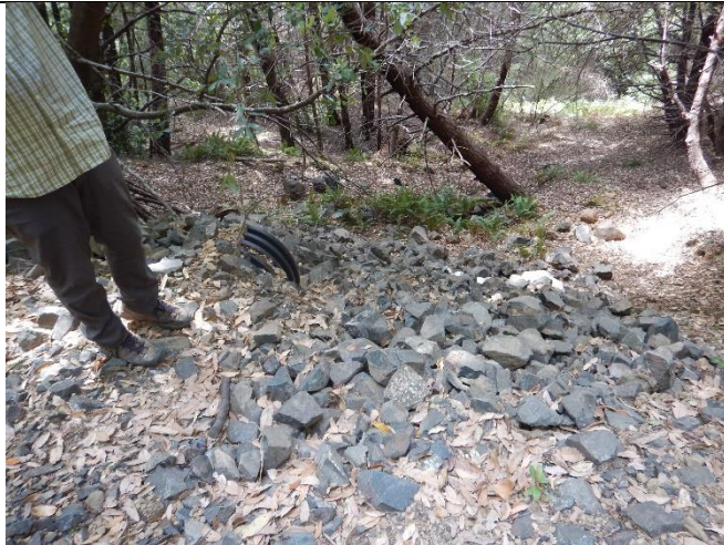
Photo 27 – FR21; culvert stream crossing outlet with rock armoring
