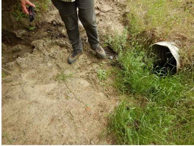
Photo 9 – FR5; inboard ditch and stream meet at culvert inlet
