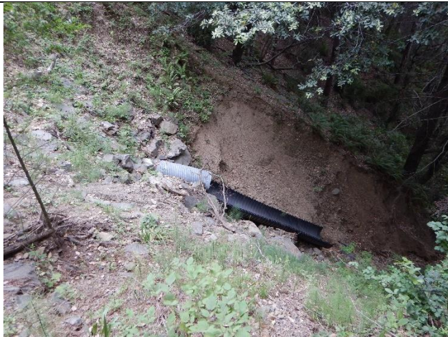
Photo 1 – FR1; inboard ditch and stream entering culvert
