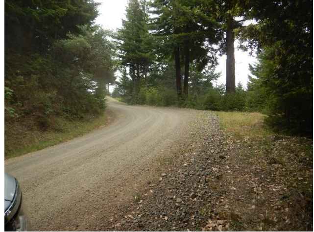
Photo 6 – FR3; insloped portion of road with inboard ditch
