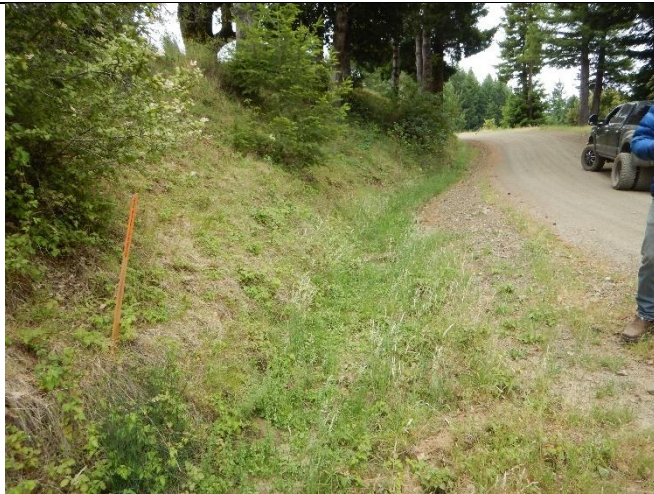
Photo 9 – FR5; inboard ditch and stream meet at culvert inlet
