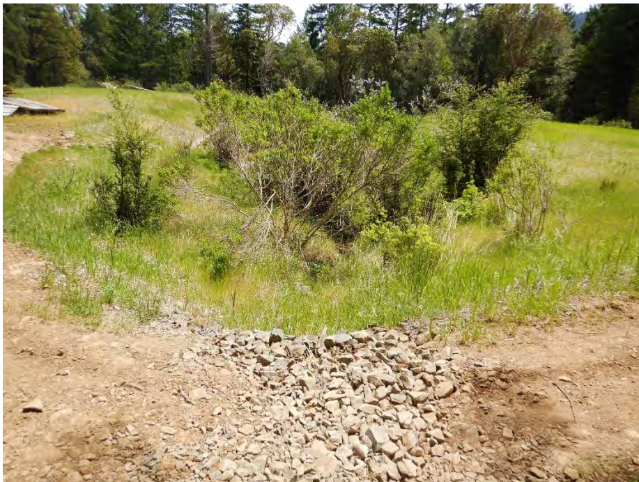
Photo 6—Rocked ford crossing at MP 24. Located north, to the left, of the area pictured in Photo 1.
