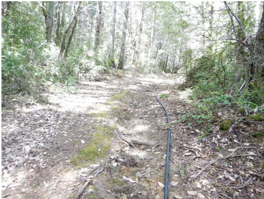
Photo 14—Looking north, uphill at rill scoured into road surface north of Map Point 20.
