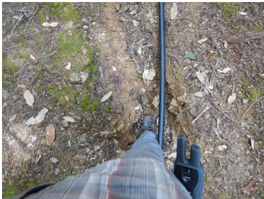
Photo 16—Looking at rill, scoured into road surface north of Map Point 20.
