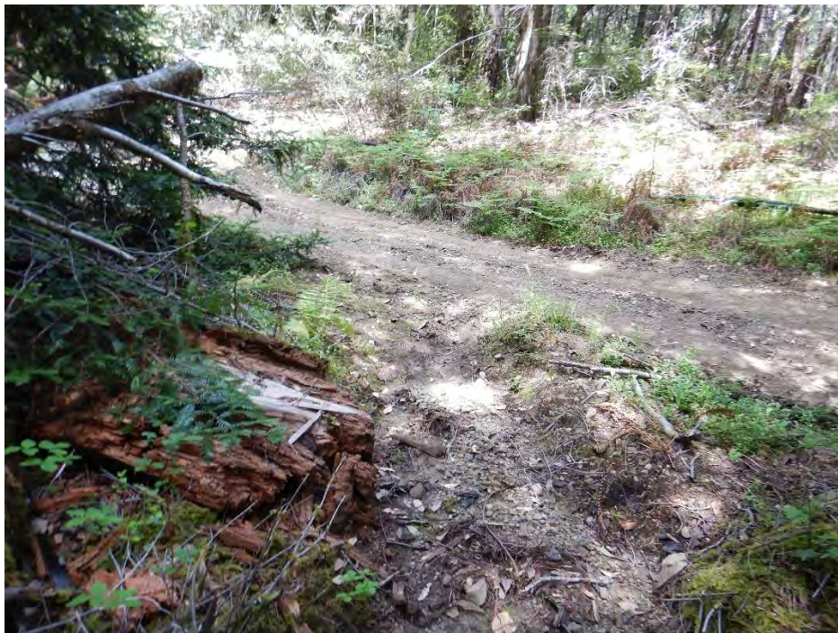
Photo 24— Looking north east in the vicinity of Map Point 18. Stormwater from the road in the upper left of the picture, would flow down the ditch where the photographer is standing before entering a watercourse behind the photographer pictured below.
