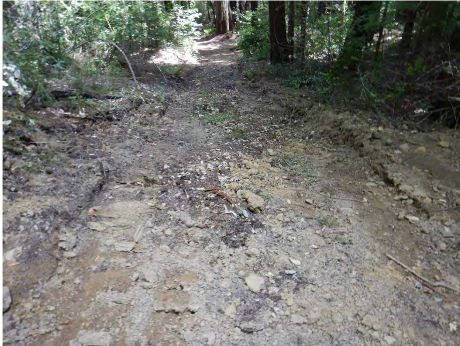
Photo 19—Tracks from recent heavy equipment use in the vicinity of Map Point 20.
