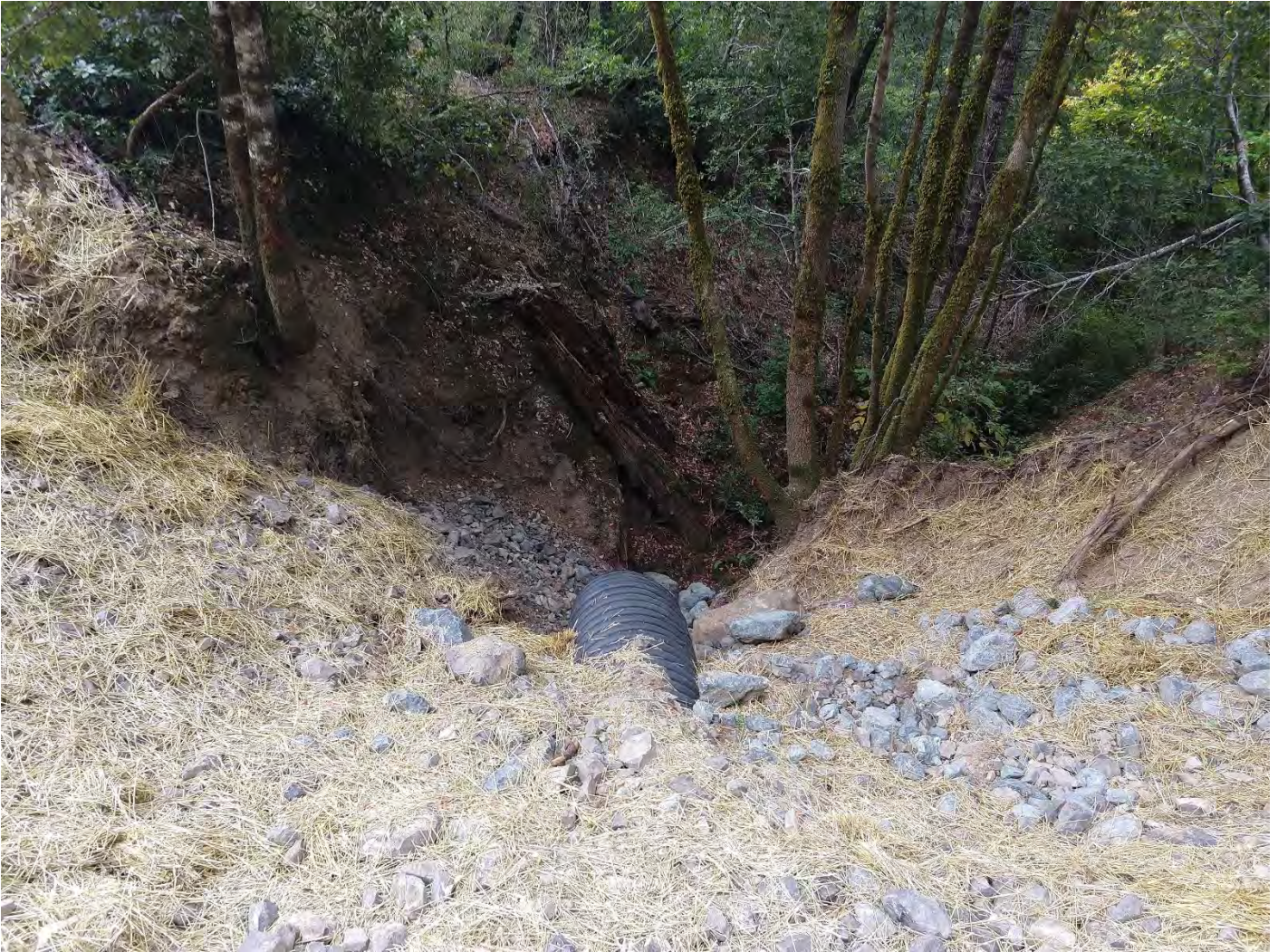
Outlet 1600 Crossing #7 (WRPP Site 08) New 30" culvert crossing adequately installed near grade with energy dissipater below outlet.
