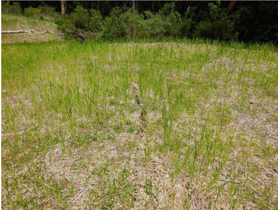
Photo 5—Tension crack in placed fill. Location identified as “crack” in Photo 1.
