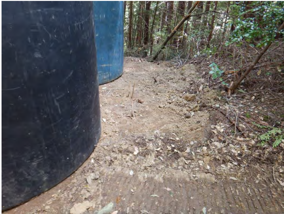
Photo 21—Tanks placed on recently constructed earthen pad in the vicinity of Map Point 20.
