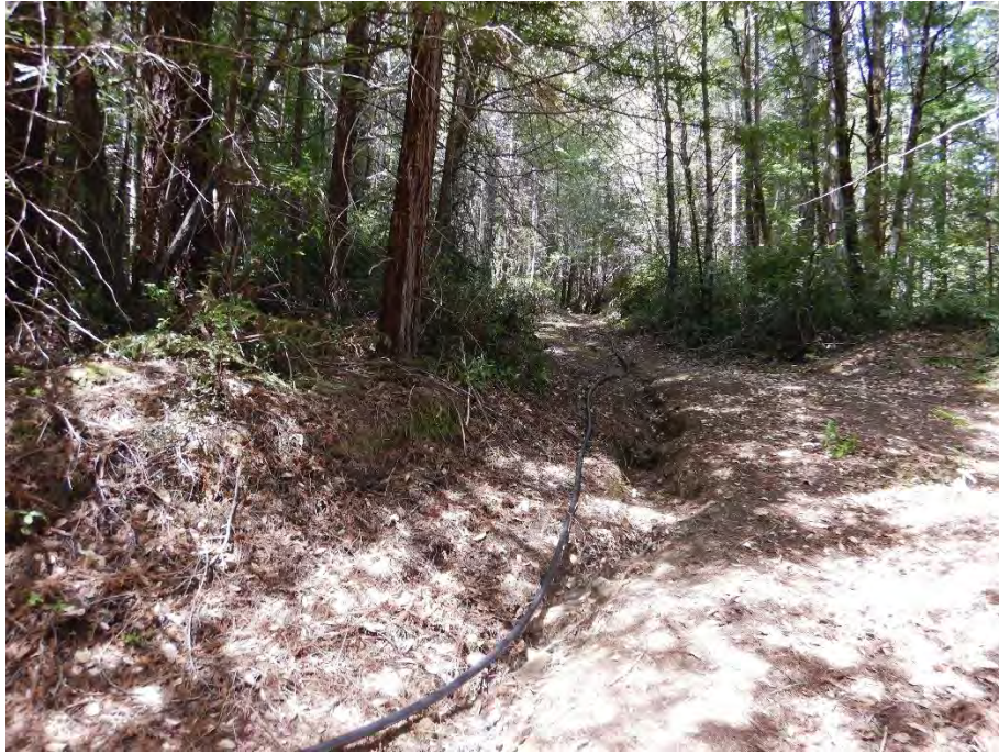
Photo 17—Looking at rill, scoured into road surface north of Map Point 20.
