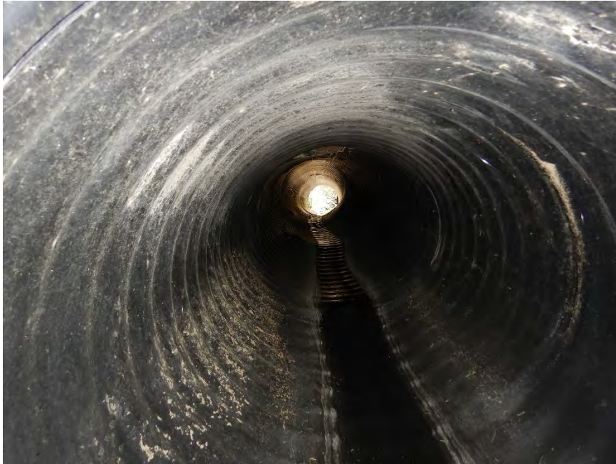
Photo 27—Looking into a 36-inch diameter culvert located at Map Point 12.
