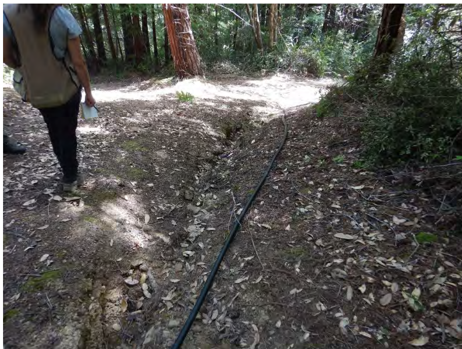
Photo 15—Looking south, downhill at rill scoured into road surface north of Map Point 20.
