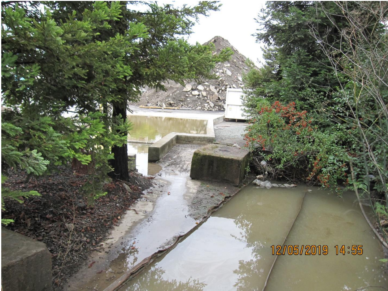
Picture 4 – View of the settling tanks and a settling pond adjacent to an asphalt recycling material stockpile – no measures in place to manage the stockpile or serve as source control. The permittee is required to ensure all minimum and advance BMPs for sediment and erosion control are implemented/ installed and maintained appropriately to eliminate or reduce the sediment that is discharged through the inlets.
