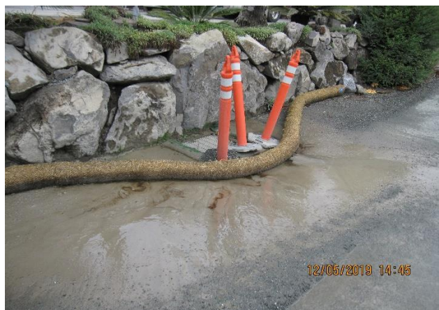
Pictures 3a, 3b – View of storm drain inlets with visible sediment accumulation and evidence of discharge of sediment into drainage system.
