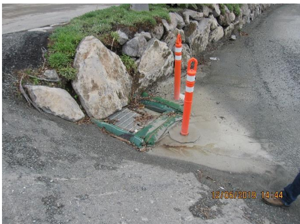
Pictures 3a, 3b – View of storm drain inlets with visible sediment accumulation and evidence of discharge of sediment into drainage system.
