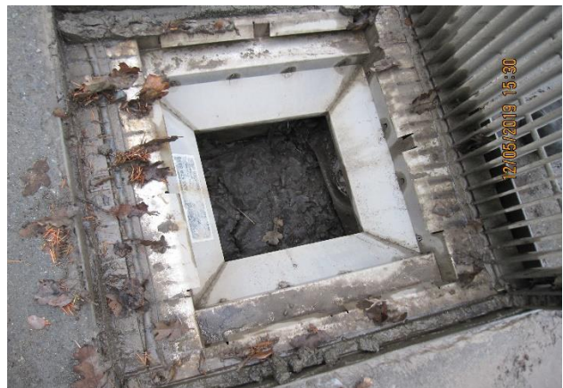
Pictures 10a, 10b – Views of unprotected drop inlet and the accumulated sediment discharged through the inlet.
