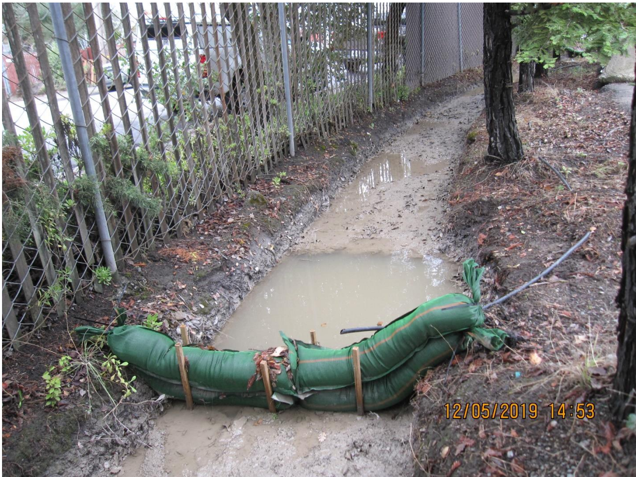
Picture 2 – View of bioswale along the southwest of the facility. Sediments trapped behind the check dams have not been removed. Significant sediment accumulation observed.
