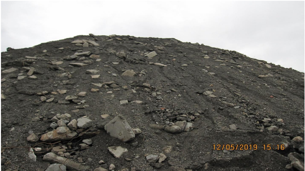
Picture 5 – View of a very large unprotected material stockpile located a few feet away from the existing muddy settling pond.
