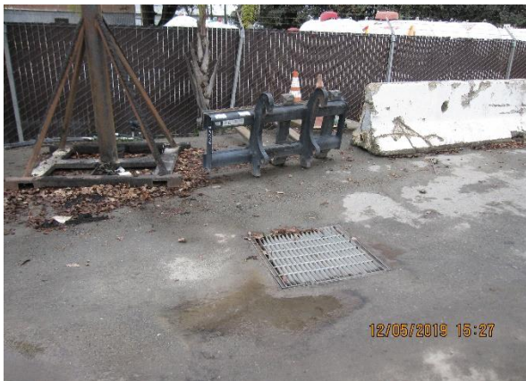
Pictures 10a, 10b – Views of unprotected drop inlet and the accumulated sediment discharged through the inlet.
