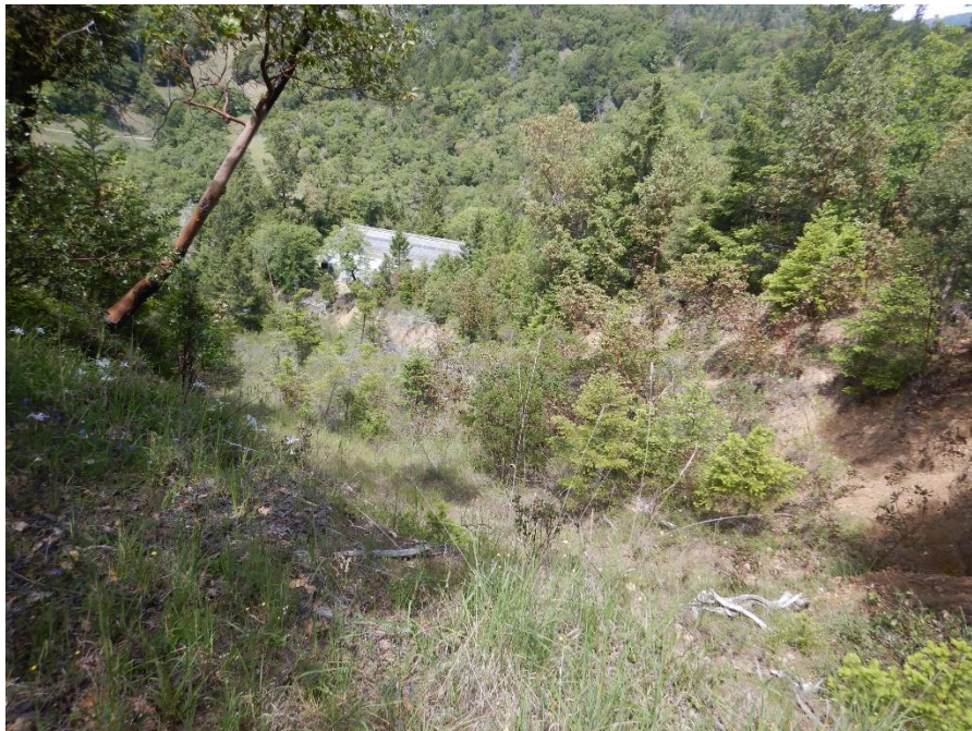
Photo 32—Looking north at landslide from landslide scarp. The Glass House at Site 1 can be seen in the middle of the image.
