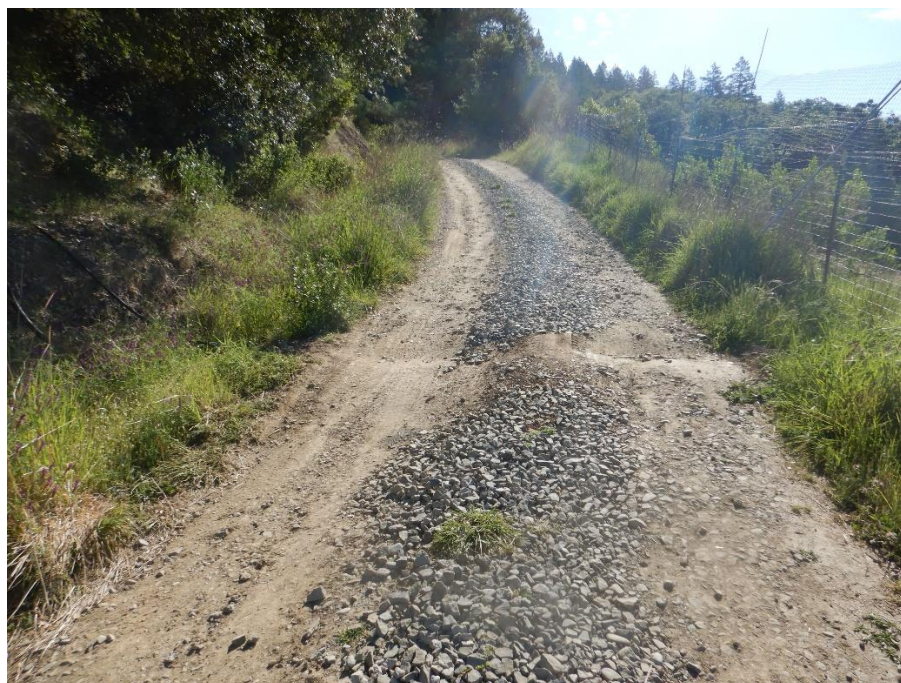
Photo 2—Looking northeast up a partially rocked road used to access Site 7 which is to the back-right of the photographer. Note small rolling dip in road at the center of image.
