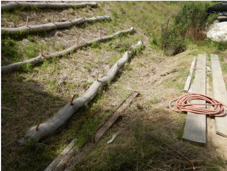
Photo 11—An earthen berm with staked wattles. The ditch at the base of the berm drains to a culvert in the back right of the image, which discharges into the watercourse running along the east side of the Glass House at Site 1.
