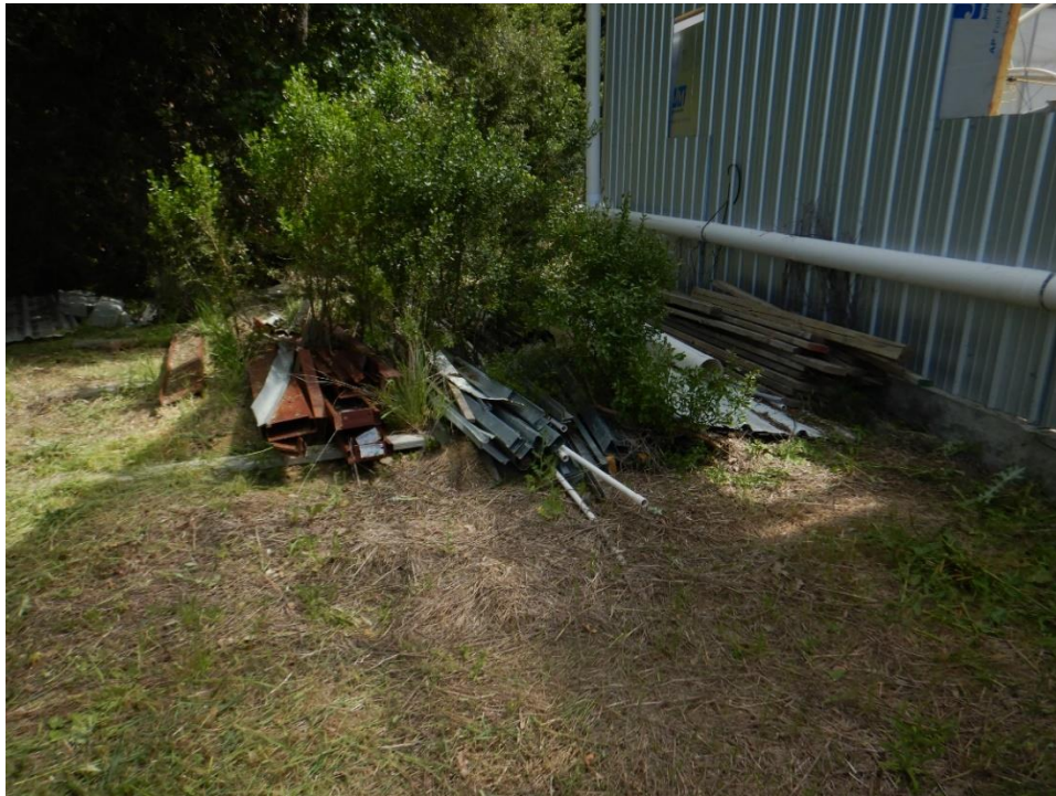
Photo 15— The northern exterior of the Glass House at Site 1. The piping strapped to the side of the building conveys stormwater collected by the roof to an area east of the pad.
