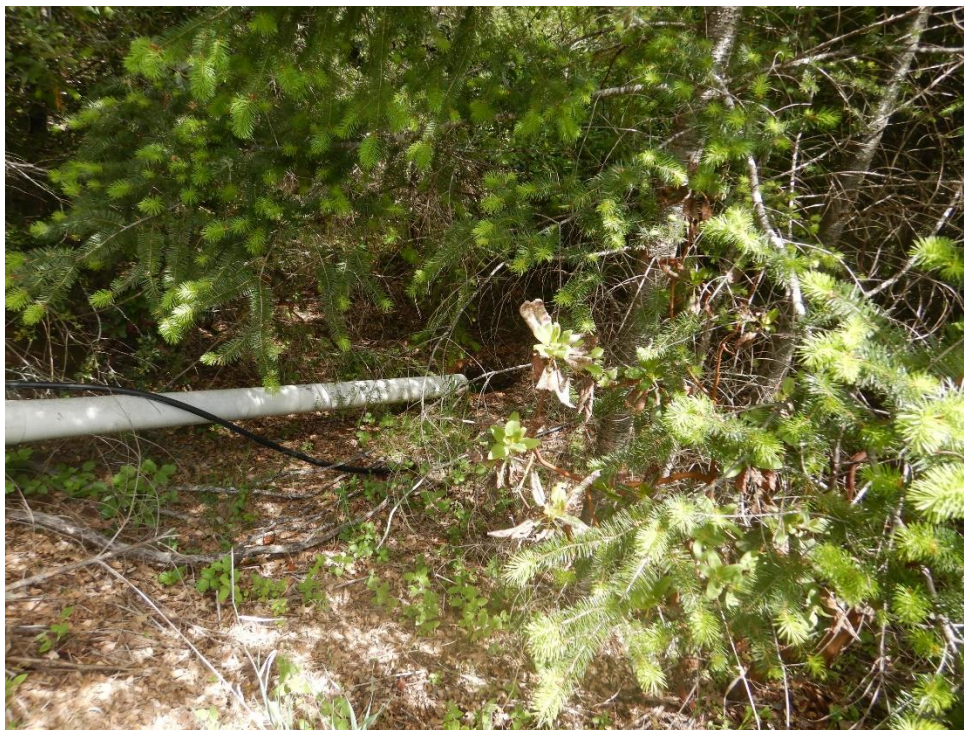
Photo 16—Discharge location of the roof gutter system pictured in previous image.
