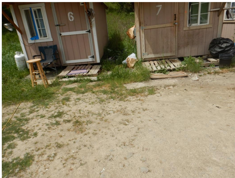
Photo 26—Looking west at second (easterly set) of small cabins. The cabins are located in the same path of stormwater as in previous years.
