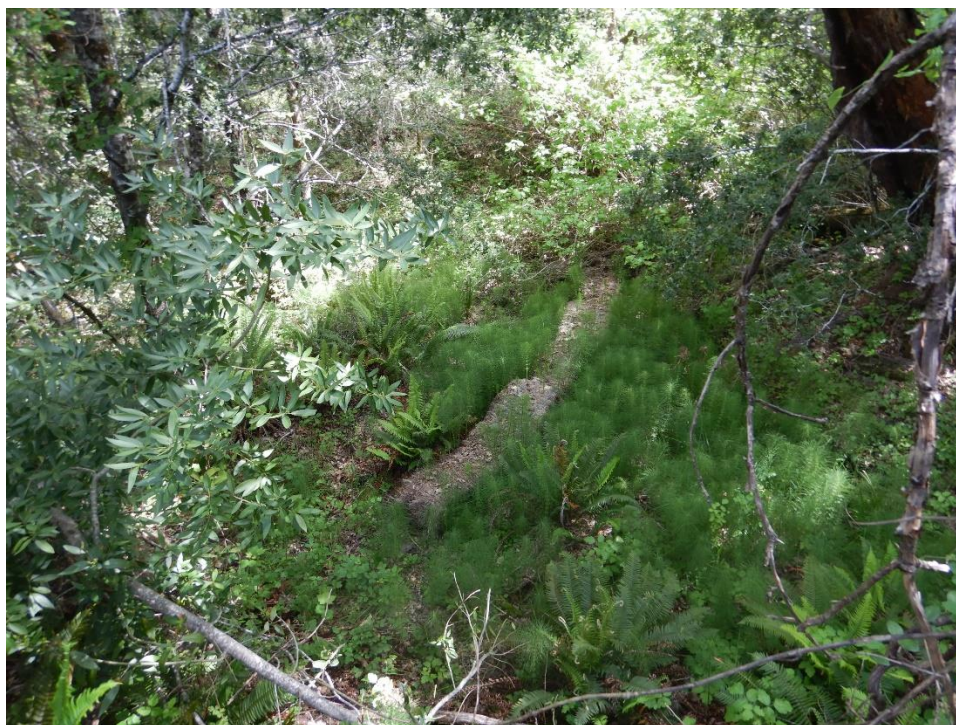
Photo 18—Hay bales installed in the sediment-filled watercourse east of the greenhouse at Site 1.
