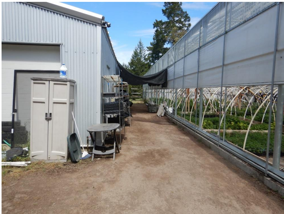
Photo 12—Shows the area west of the Glass House at Site 1.
