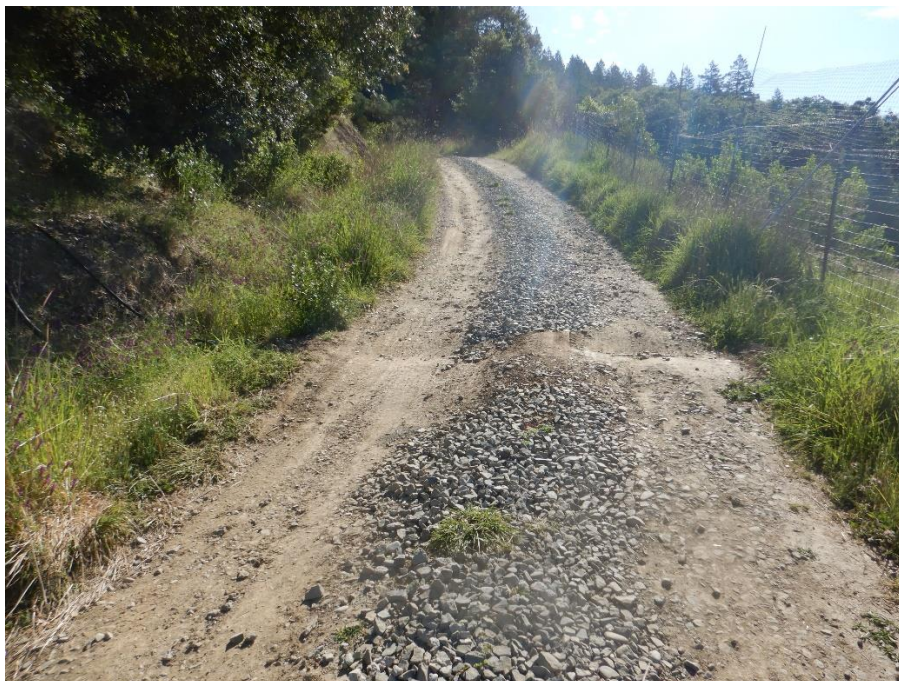
Photo 2—Looking northeast up a partially rocked road used to access Site 7 which is to the back-right of the photographer. Note small rolling dip in road at the center of image.
