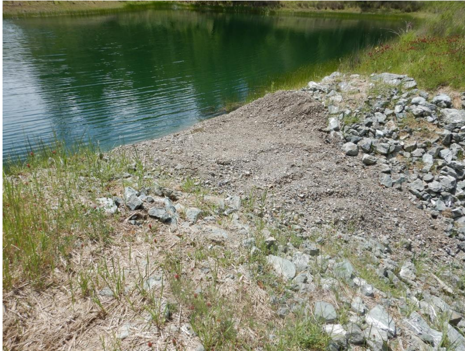
Photo 19—Looking west at the Reservoir weir. The overflow is composed of fine gravel.
