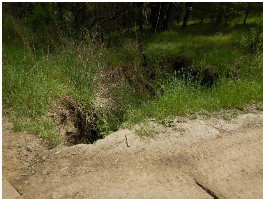
Photo 24—The watercourse downstream from the access drive pictured in the previous image. Note the watercourse is deeply incised.
