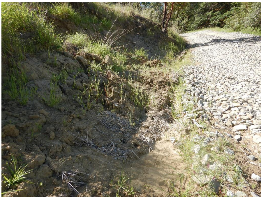
Photo 1—Looking east along the road accessing Site 7. Dried clumps of earth on road's cut-bank suggests water continues to seep seasonally from the area from a watercourse that infiltrates the earthflow material to the left of the image.
