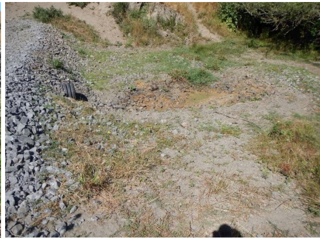
Culvert outlet center left. Some bed scour erosion below outlet.
