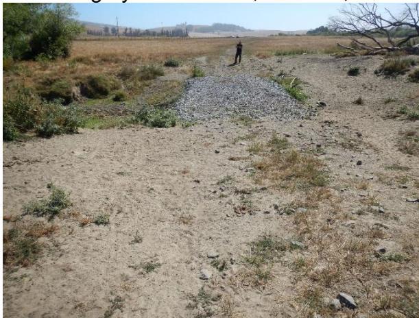
Watercourse crossing of Americano Creek – subject of complaint.
