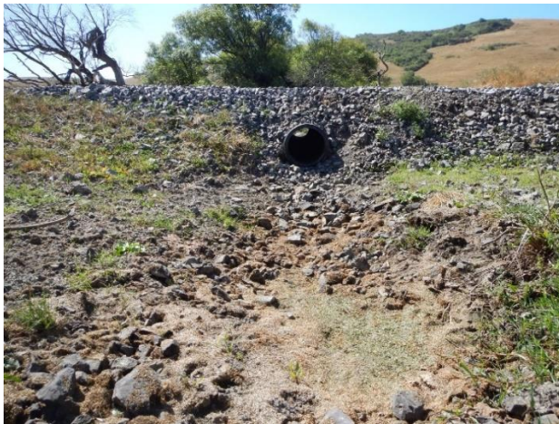
Culvert outlet area.
