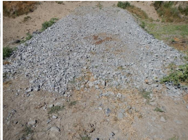
Close-up of crossing. Note angular rock used.
