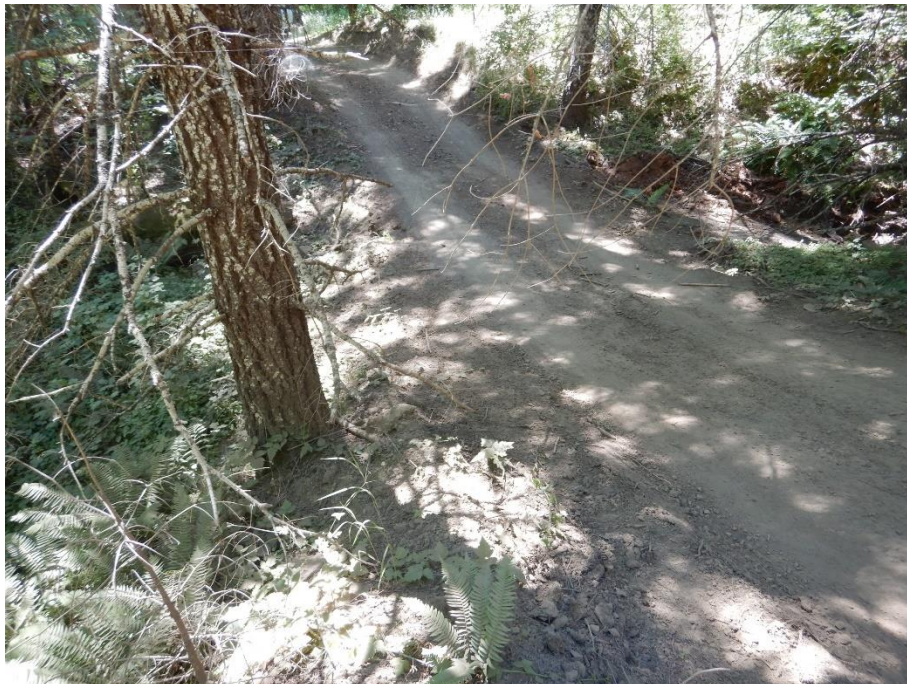
Photo 20—Looking at the road crossing a watercourse at WQ 10. The road does not have any road aggregate to prevent erosion and the road shape does not provide a path for stream overflow outside from the road fill.
