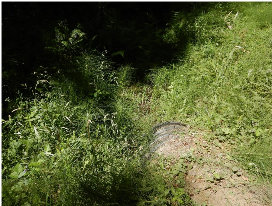
Photo 14— Looking upstream at a 24-inch diameter culvert at WQ 7. The watercourse upstream is approximately four feet wide.
