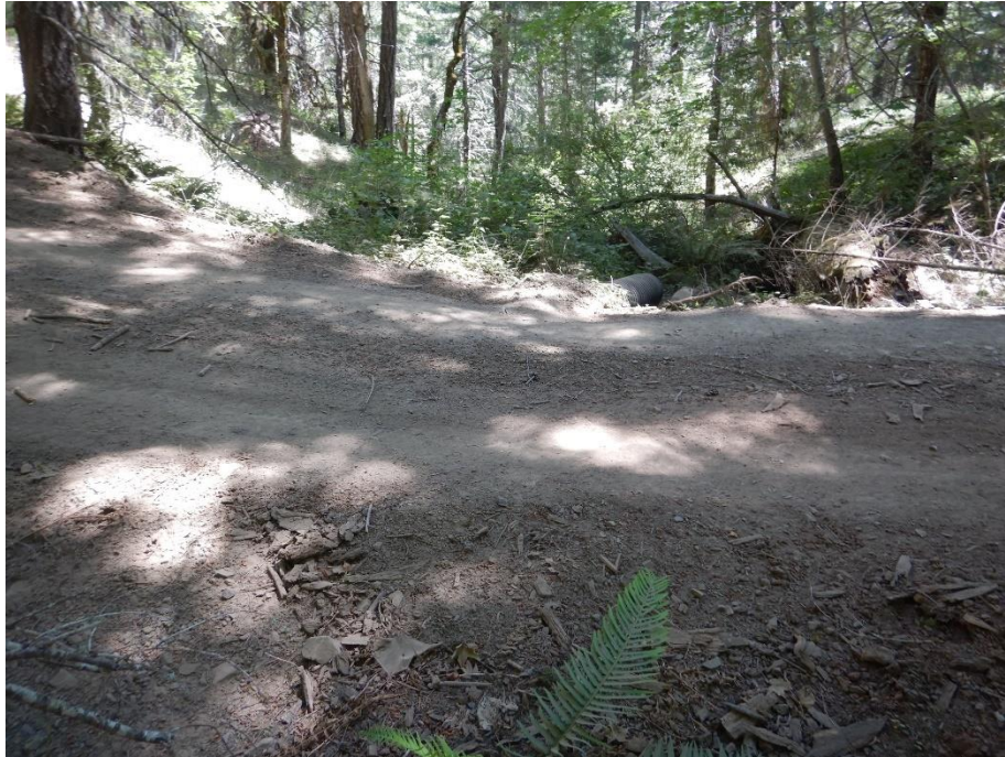
Photo 21—Looking downstream at WQ 10. The culvert is only partially buried in the road fill prism.
