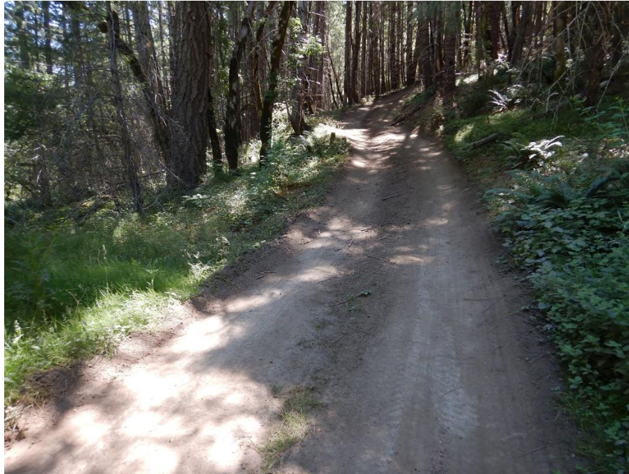
Photo 15— Looking east along a dirt road approaching the stream crossing at WQ 8 which is behind the photographer. The road is steep and lacks features, such as water bars or rolling dips, to direct stormwater off the road. The road's earthen surface is susceptible to erosion by stormwater.
