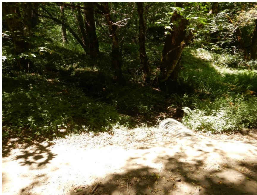
Photo 16— Looking upstream at a 24-inch diameter culvert at WQ 8. The watercourse upstream is approximately four feet wide. The culvert is only partially buried in the road fill prism.
