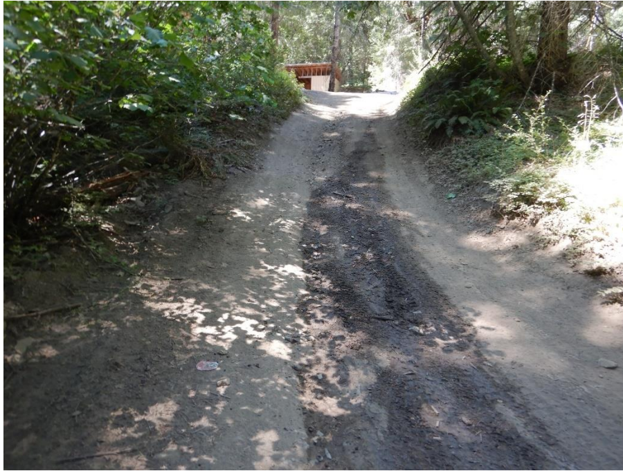
Photo 13—Looking south along a dirt road towards the shed pictured in Photo 11. The road is steep and lacks features, such as water bars or rolling dips, to direct stormwater off the road. The road's earthen surface is susceptible to erosion by stormwater.
