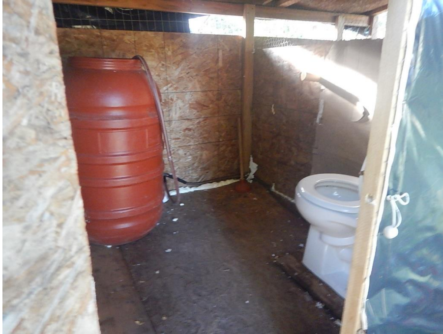
Photo 1—Taken June 27, 2019, flush toilet located at WQ 1.
