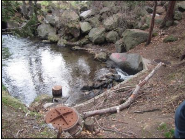
Photo 5: View looking southwest of the manhole adjacent to Boles Creek.
