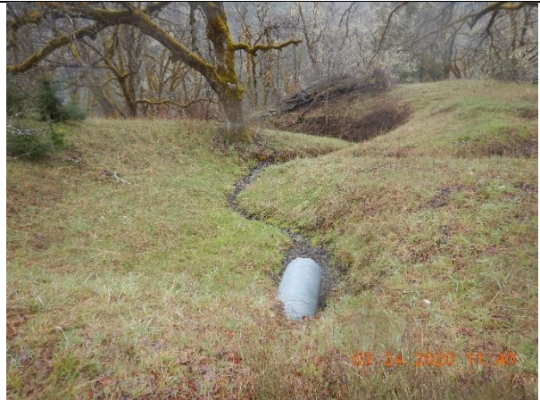
Photo 14 – Culvert stream crossing
