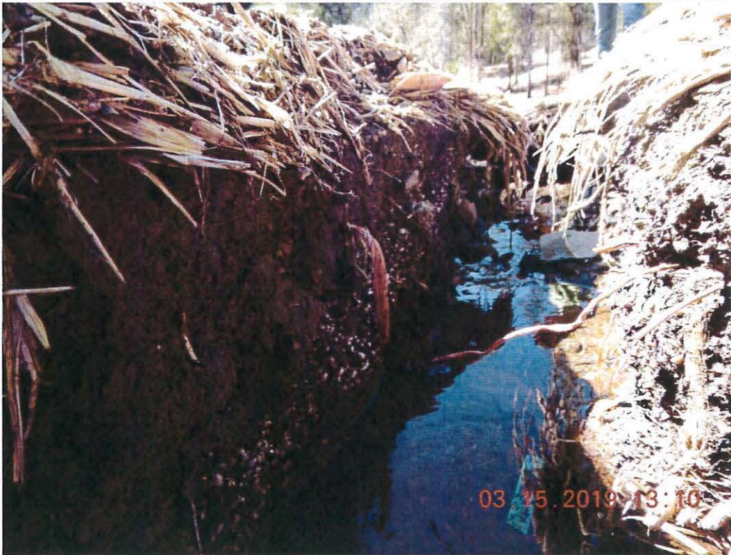
Figure 3. Examples of the stream cutting through placed fill, potting soil, and trash; depth of incision ranged from a few inches to over a foot. Note the layer of potting soil.
