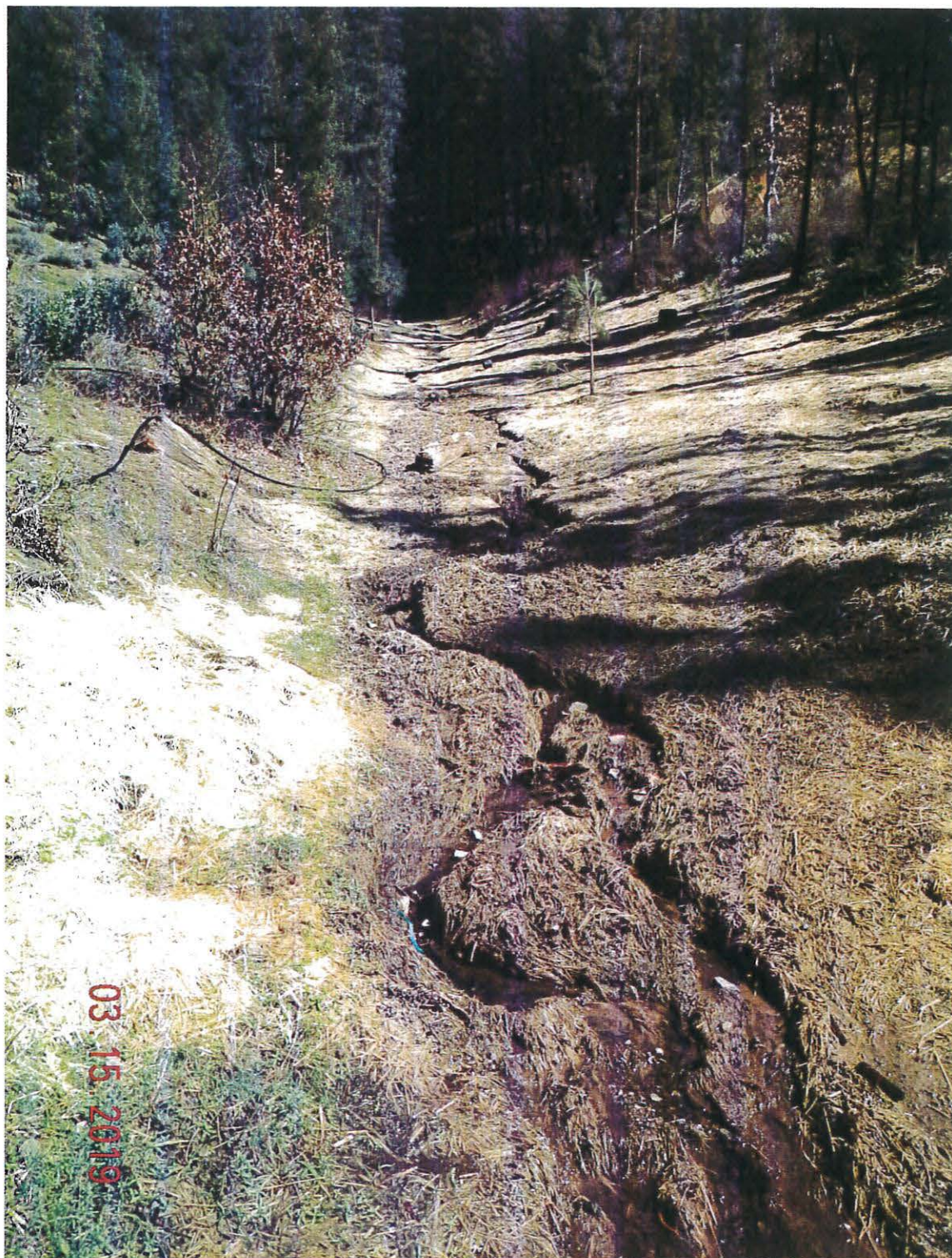
Figure 1. Unnamed stream tributary to Salt Creek where alteration, sediment and nutrient discharges, and trash were documented. Approximately 275 feet of the stream was graded and altered. Note the algae in the foreground, likely due to elevated nutrient levels from potting soil and fertilizers.
