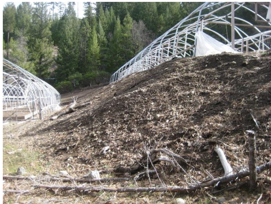
Western side of GH2 flats looking east. Note scale of fill.
