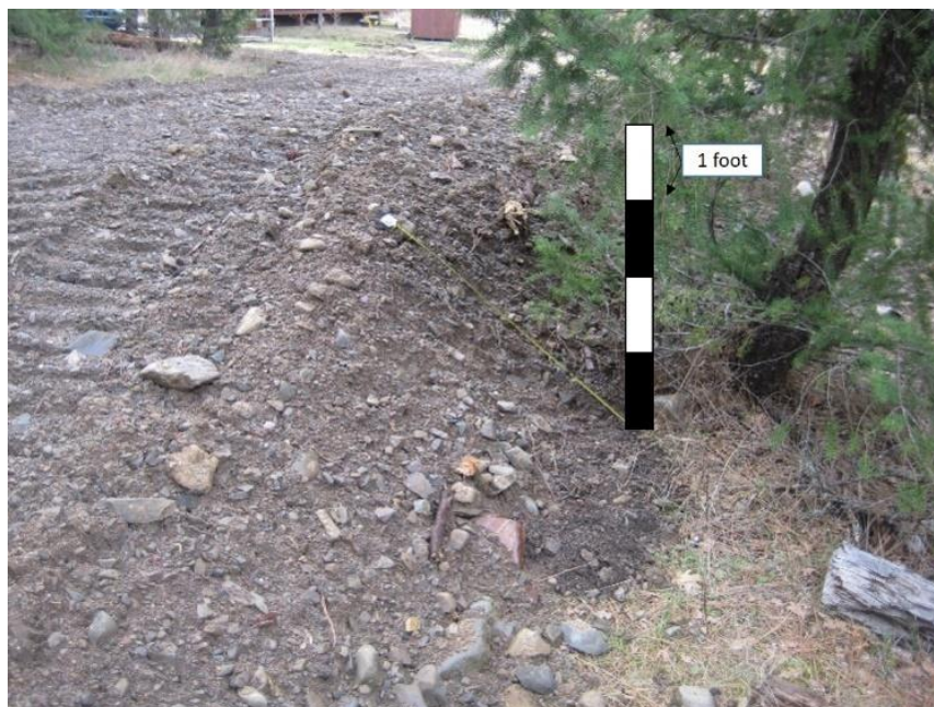
Photo taken at northeastern edge of NGA looking southwest. Annotated scale shows ~4 foot depth of fill.
