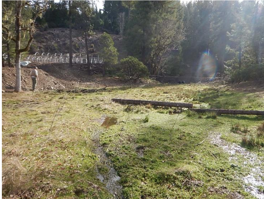
Photo looking east towards GH1 (upper left portion of image) from suspected wetland at downstream end of newly constructed crossing.
