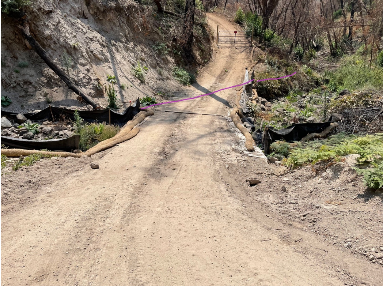
Figure 4. View of crossing taken from the west side of crossing. Purple line shows approximate location of bankfull depth of channel.
