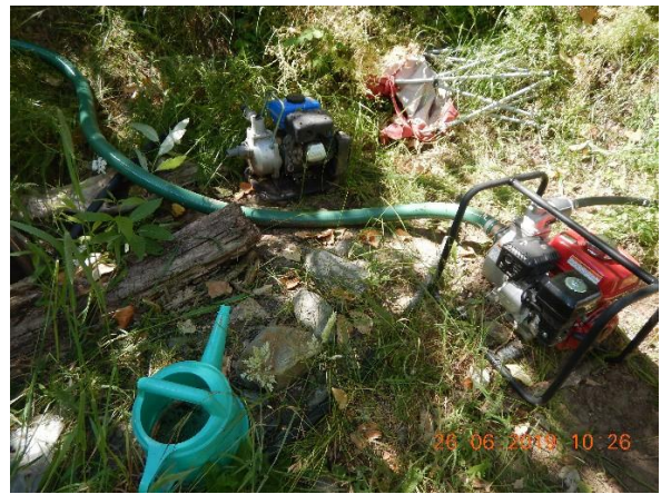
Photo Taken by: Pansy Yuen, 26 June 2019 Photo 62 – Close-up view of a water pump connected to a green suction hose stored behind the corrugated riser pipe.
