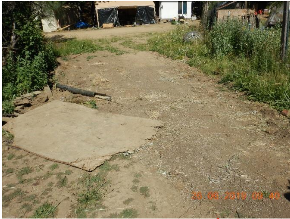
Photo Taken by: Pansy Yuen, 26 June 2019 Photo 37 – West view of fill in a Class III watercourse.
