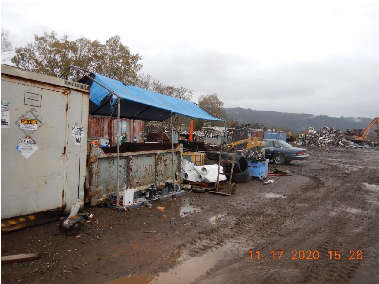
Picture 2 – View of non-watertight dumpster that is being placed on the ground with an inappropriate cover. Picture taken by Farzad Kasmaei.
