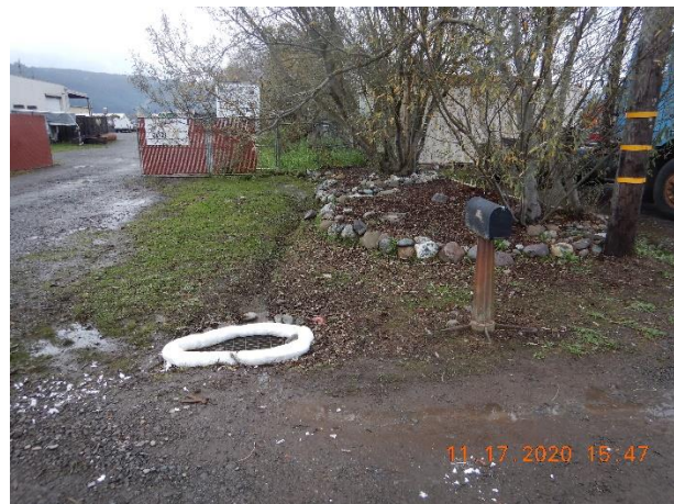
Pictures 9a, 9b – Views of sampling point on the northwest side of the facility adjacent to the main office. The samples are collected from a shallow trench where the runoff leaves the site on its way being discharged into an off-site drop inlet (DI). DI is protected with an absorbent sock. Site Map:
