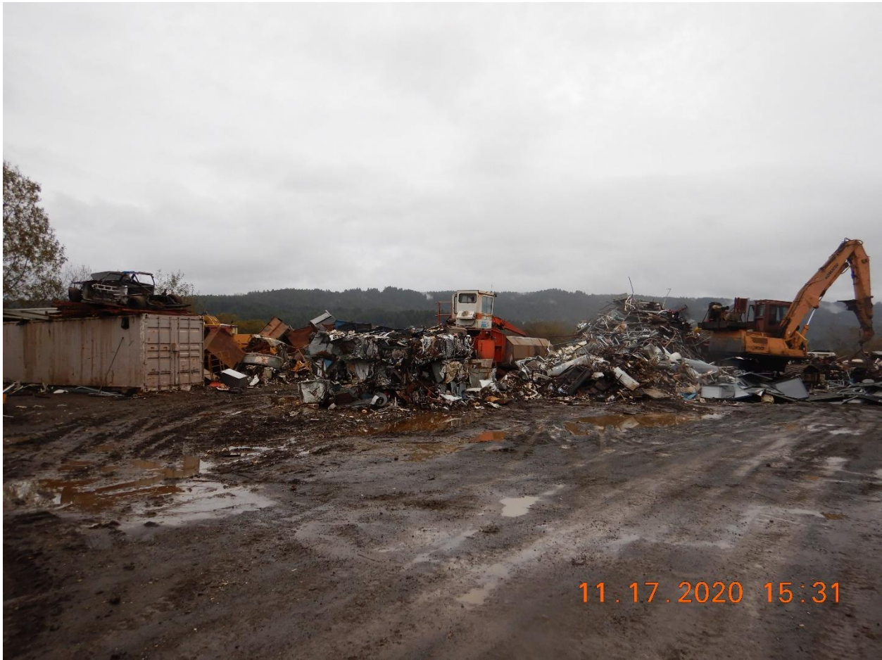
Picture 4 – View of a huge scrap metal stockpile stored directly on the ground and exposed to rain. No BMPs implemented/installed throughout the facility to eliminate or at least minimize the exposure of industrial material/equipment to rain.
