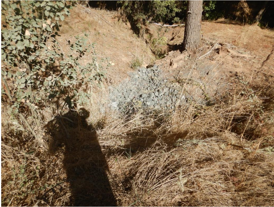
Photo 3—Outlet to reservoir outfall located at WQ 2.
