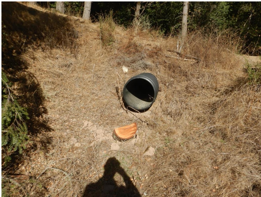
Photo 2—Inlet to reservoir outfall at WQ 2.
