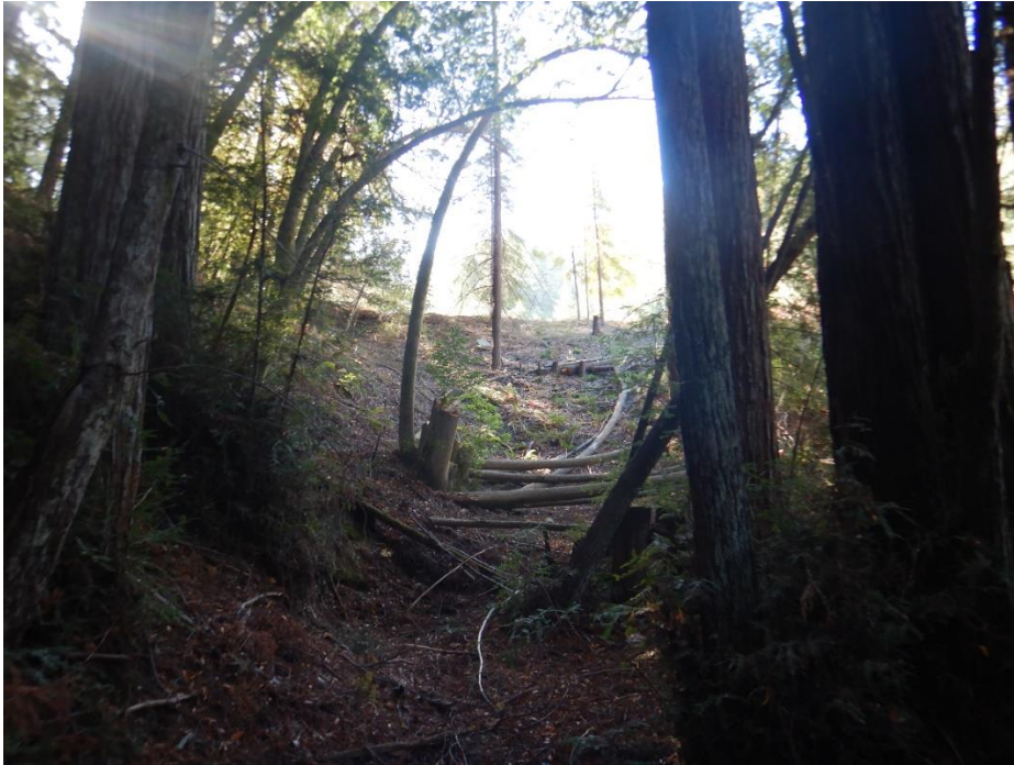
Photo 17—Looking towards dam embankment where previous photo was taken from. Cistern at WQ 9 is to the back of the photographer.
