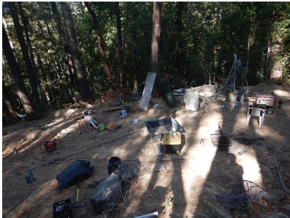
Photo 10—Showing work area for uncompleted groundwater well at WQ 7.
