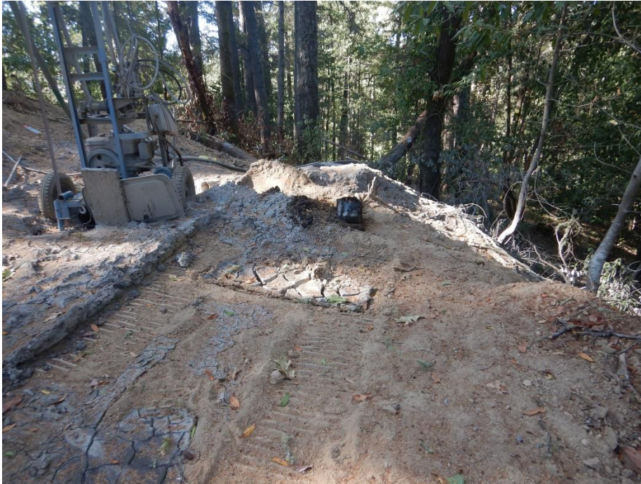
Photo 11—Drill rig and open bucket with black substance at WQ 7.
