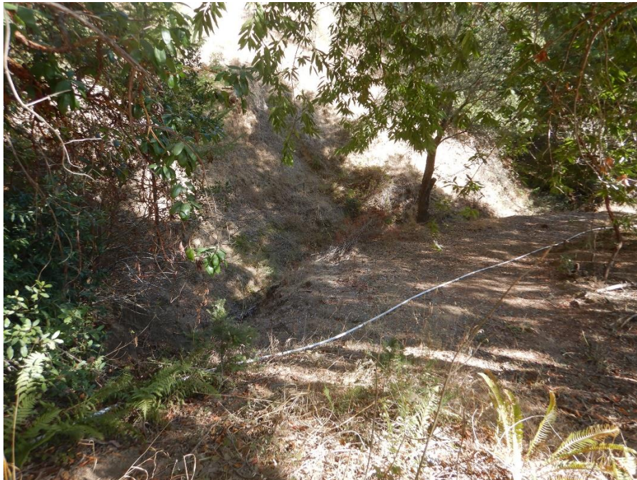
Photo 1—Historical road encroaching on a watercourse at WQ 1.
