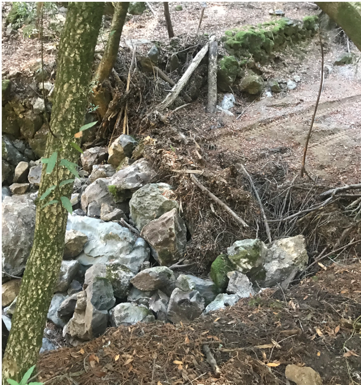
Figure 3 Earthen fill and rocky debris in channel of Felta Creek in violation of California Water Code and Federal Clean Water Act.
