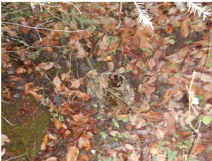
Photo 28—Looking west and downstream at inlet of a 15-inch diameter metal pipe located at WQ 17.
