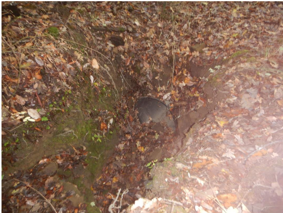
Photo 34—Inlet of an 18-inch diameter culvert at WQ 21.
