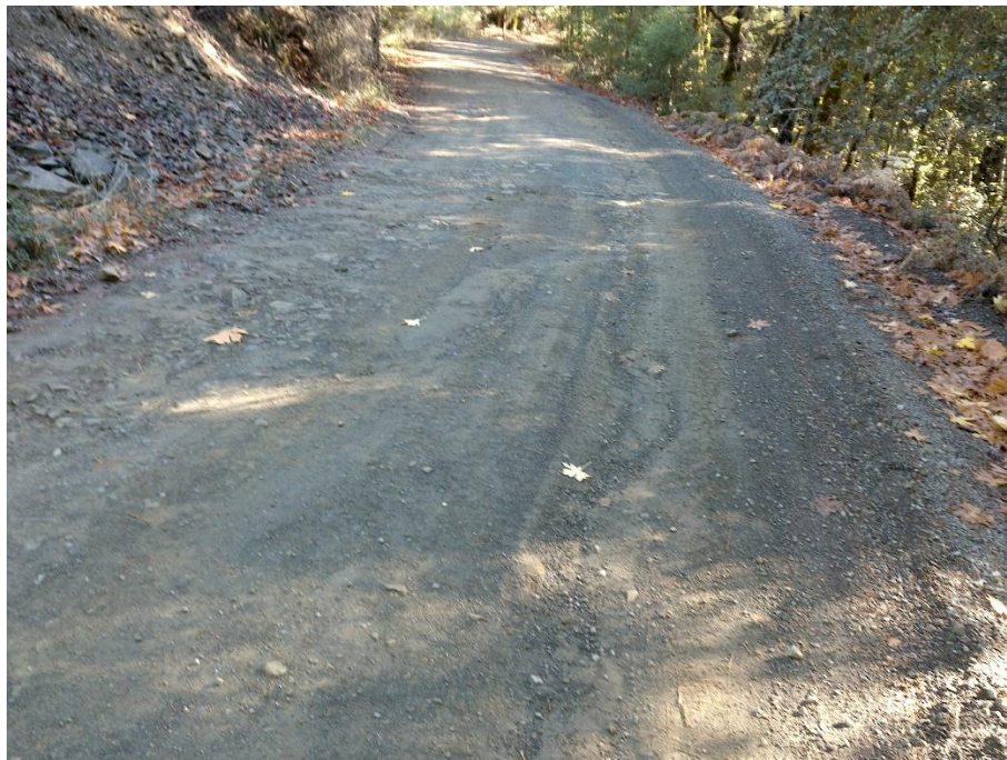
Photo 32—Looking east at road surface in the vicinity of WQ 19. From this location, stormwater is collected by the road and transported in an inboard ditch before leaving the road at WQ 20 pictured below.
