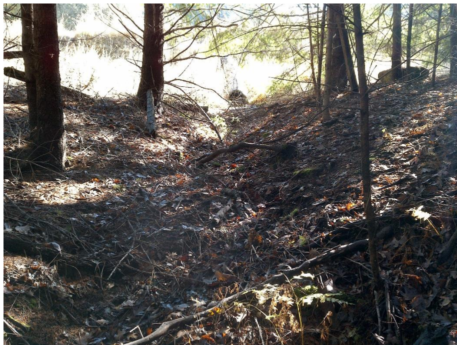
Photo 18—Looking upstream towards the reservoir outfall at WQ 11
