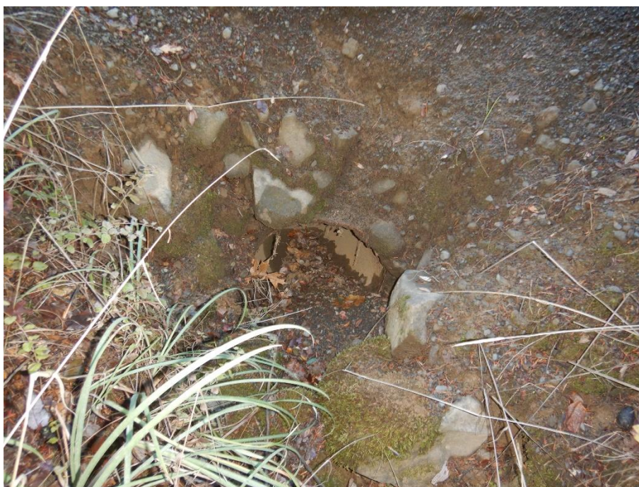
Photo 30—Looking west and downstream at inlet of an 18-inch diameter culvert located at WQ 18.
