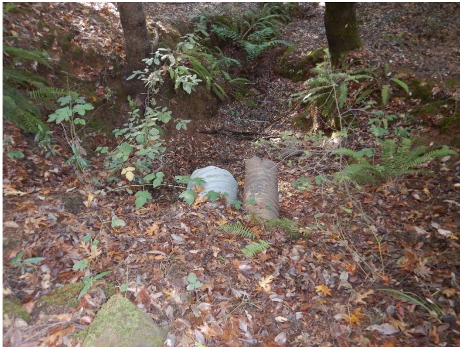
Photo 26—Looking downstream at two culverts, 12 inch and 18 inches in diameter, directed to an approximately five-foot-wide watercourse at WQ 16.
