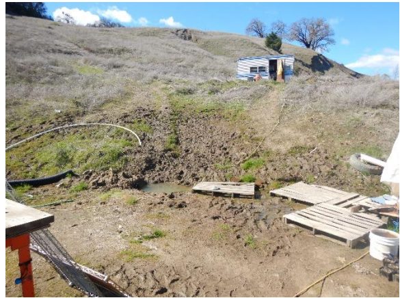
Figure 27. Standing water and flexi pipe in ditch northern cutbank of the flat.
