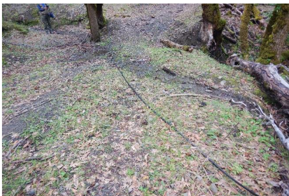
Figure 38. Diverted watercourse due to plugged culvert.
