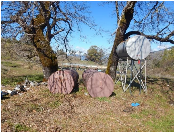
Figure 8. Fuel tanks are located under the big oak tree, as see in Figure 4, approximately 18 feet from the centerline of the watercourse.
