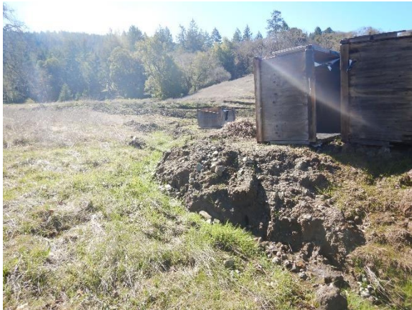
Figure 9. Fill is pushed in the watercourse at the cultivation flat.
