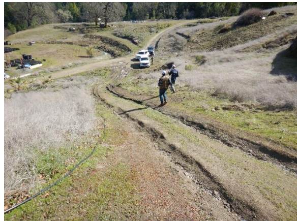
Figure 12. A steep unsurfaced road deliver sediment via rills and stormwater, to the watercourse in Figures 10 & 11.
