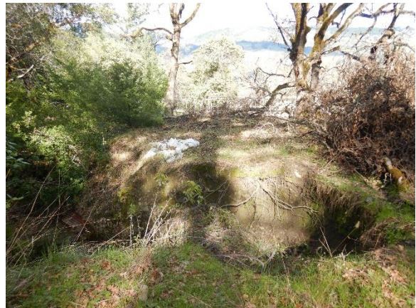
Figure 34. Eroded watercourse crossing, from left bank, looking downstream.
