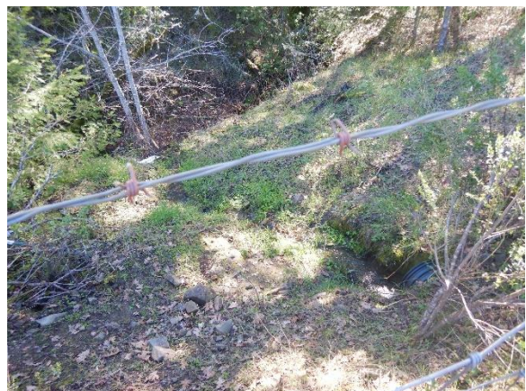
Figure 17. View of Pond 2 outlet pipe discharging to watercourse.
