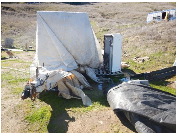
Figure 26. Generator stored next to standing water shown in previous figure.
