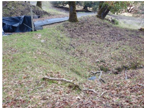
Figure 35. Water bladder located adjacent to stream crossing lacks containment.
