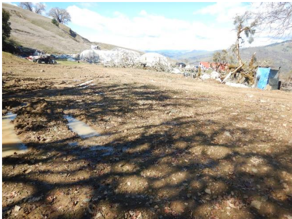
Figure 32. South of the cultivation flat has recent grading; I did not observe significant cut or fill slopes.
