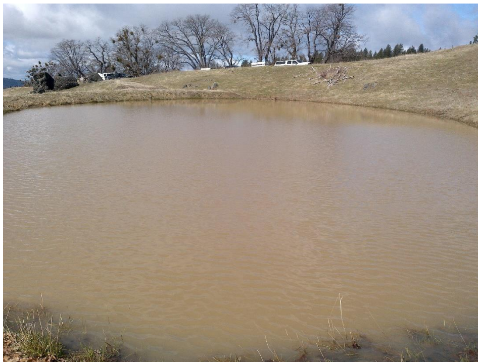
Photo 27—Looking north at reservoir (Reservoir No. 3) located at WQ 8.
