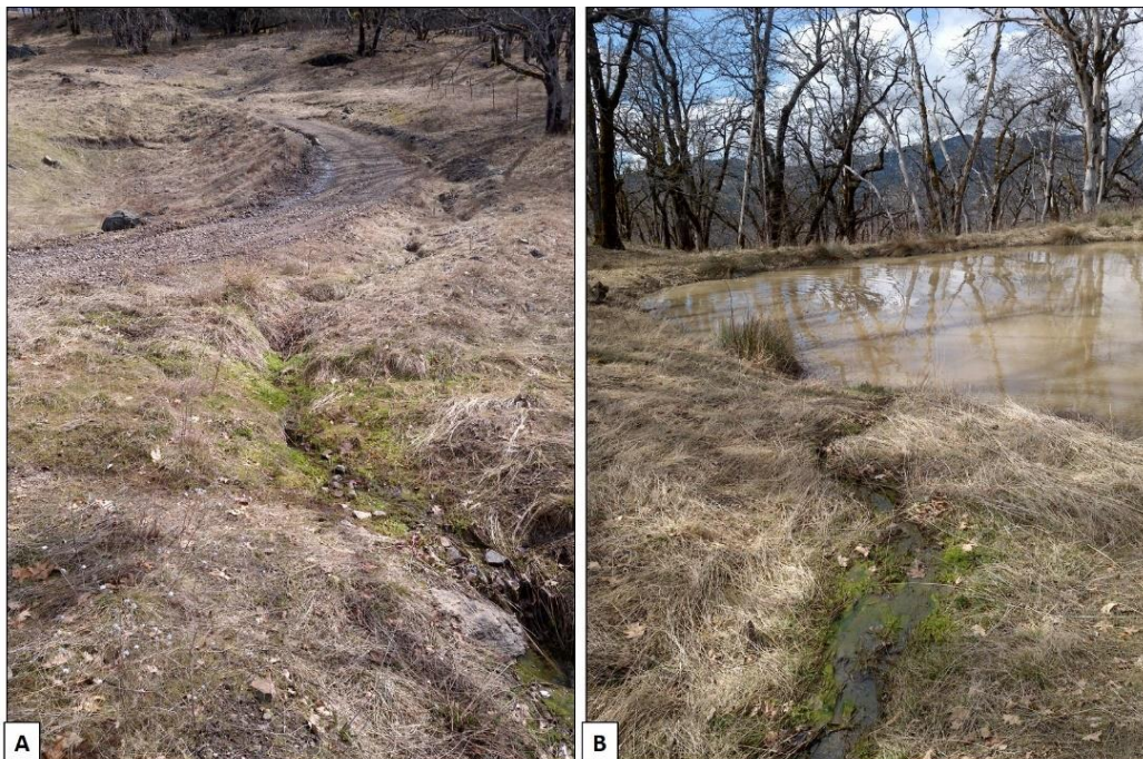
Photo 19—Looking (A) east at watercourse bordering south side of road and (B) west where watercourse enters Reservoir No. 2.
