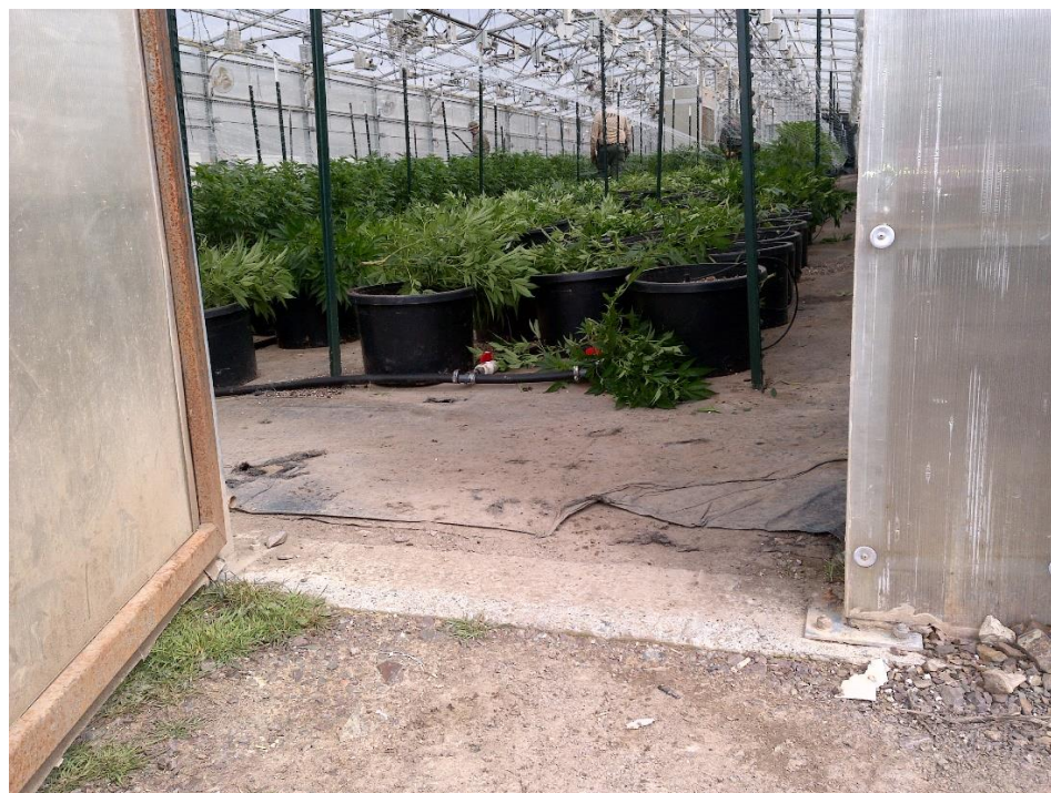
Photo 23—Greenhouse in the vicinity of WQ 7. The greenhouse floor is composed of a geotextile fabric covering dirt.
