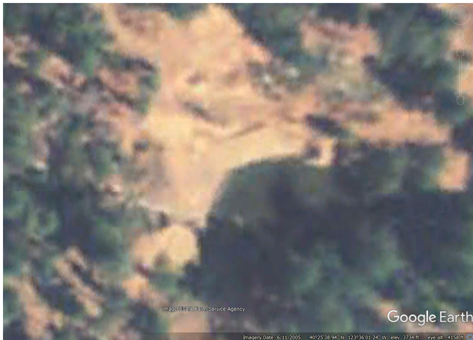
Aerial Image 3—dated June 11, 2005, accessed with Google Earth. Image shows a depression on the downstream buttress of Reservoir 1, suggesting it had failed.
