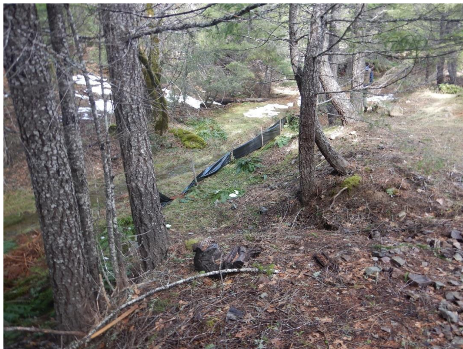
Photo 3—Silt fencing bordering watercourse south of WQ 2.
