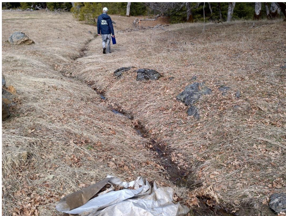
Photo 26—Looking at watercourse within 20 feet of disturbed area associated with the greenhouse at WQ 7. The greenhouse is to the left of the photographer.
