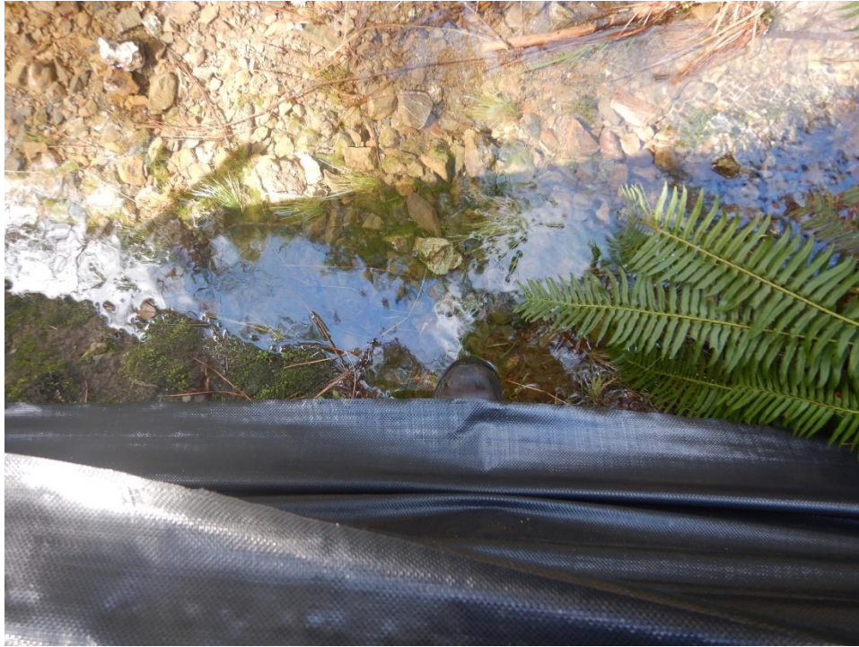
Photo 4—A boot poking under silt fence south of WQ 2.
