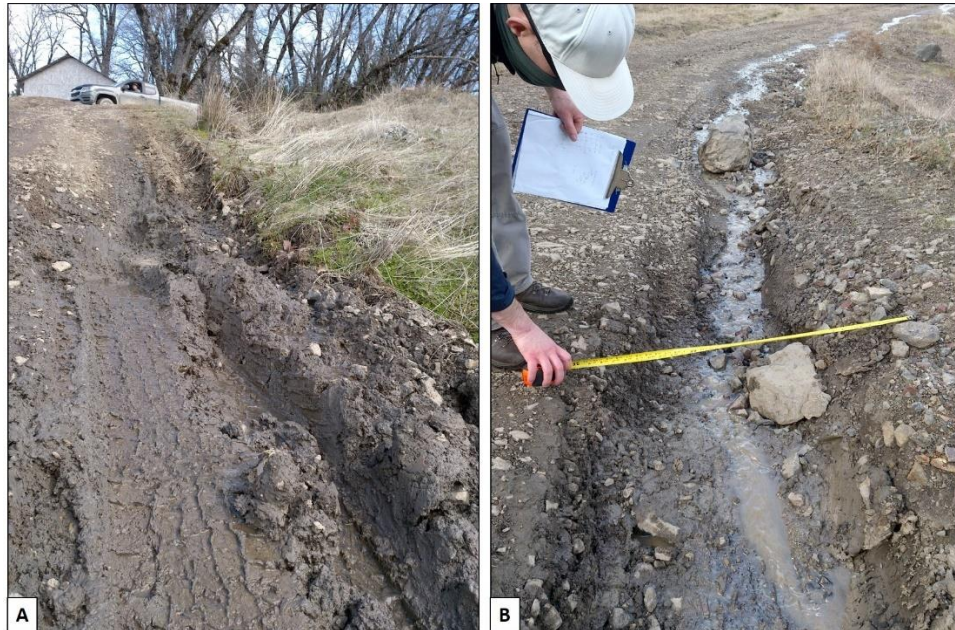
Photo 20— (A) Water emanating from a ground seep at WQ 6 and (B) flows in road channel that continues to watercourse entering Reservoir 2 pictured in Photo 19.
