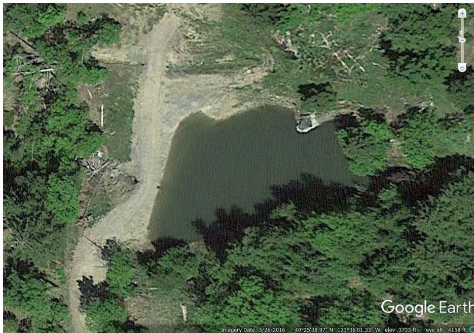
Aerial Image 9—dated May 26, 2016, accessed with Google Earth. Image shows a culvert installed in the channel fully crossing the downstream buttness of Reservoir 1.
