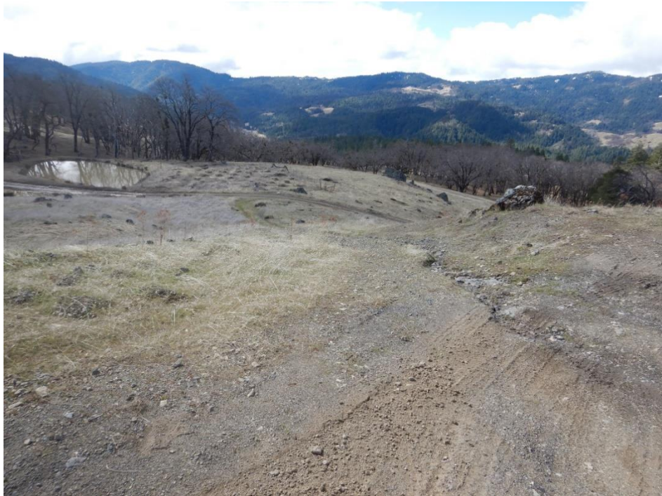
Photo 17—Looking south. The greenhouse pad at WQ 4 is to the photographer's back. A reservoir is visible in the back left of the image at WQ 5 (Reservoir No. 2). Rills are visible on the road-surface to the right of the image.
