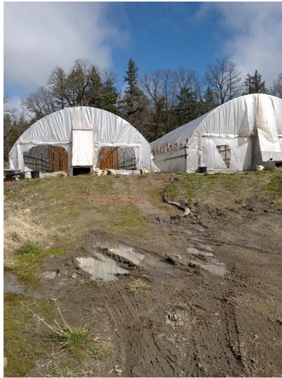
Photo 16—Looking north at pooled water at the south side of the greenhouse pad located at WQ 4.
