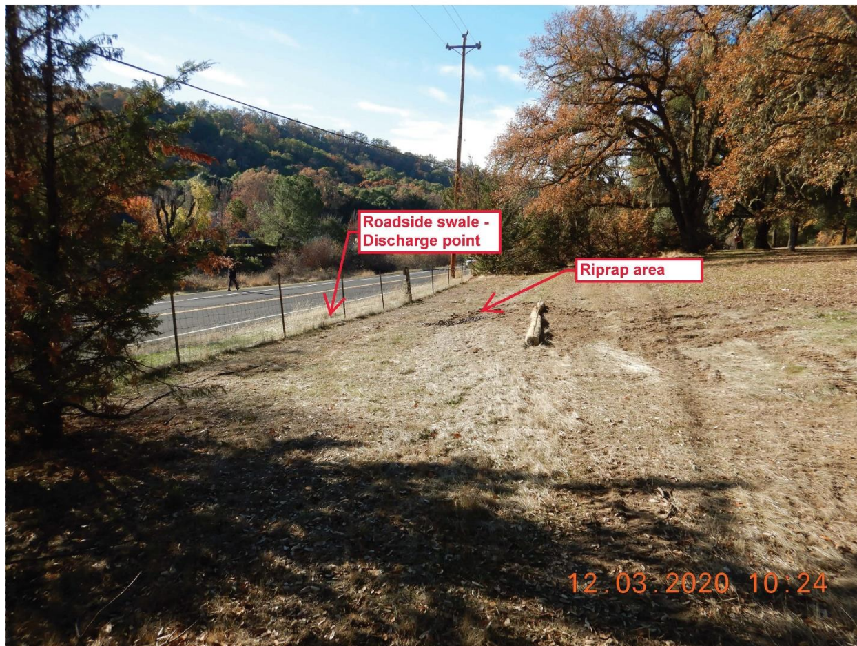
Picture 11 - View of sampling point No. 3. The samples are collected from the small riprap area down gradient of the wattle shown in the picture. Runoff to this discharge point is not concentrated, but rather is anticipated to sheet flow from DA-3 to the approximate location shown. Picture taken by Farzad Kasmaei.
