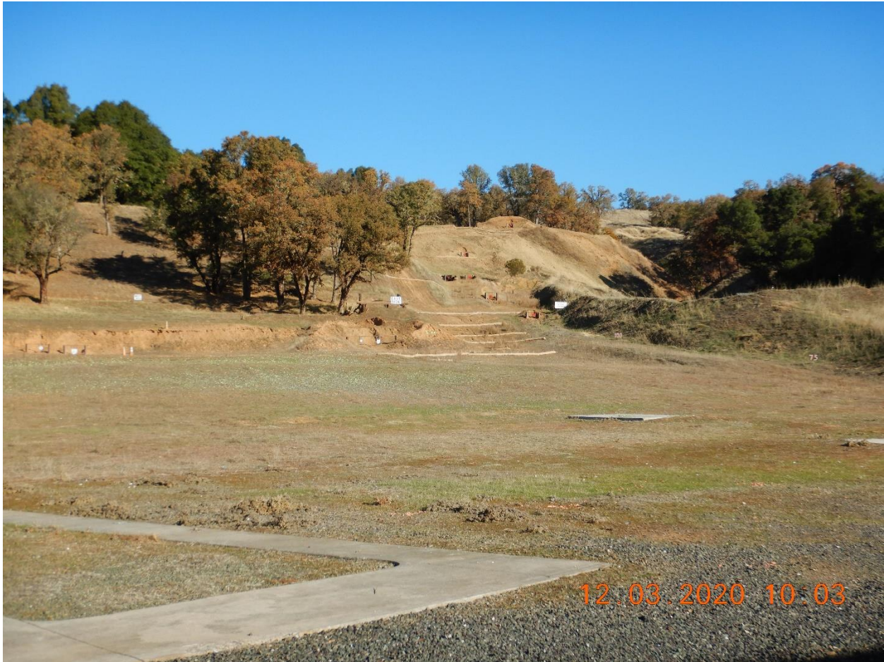
Picture 9- View of the northeast corner of the main range area where several fiber rolls are installed for sediment/erosion control. Located in DA-2 Picture taken by Farzad Kasmaei.
