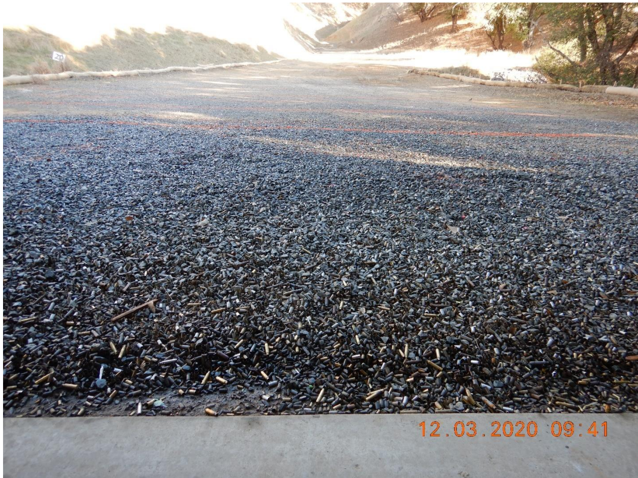
Picture 1- View of the shooting area in DA-1. Fiber rolls installed as a perimeter control BMPs. Picture taken by Farzad Kasmaei.
