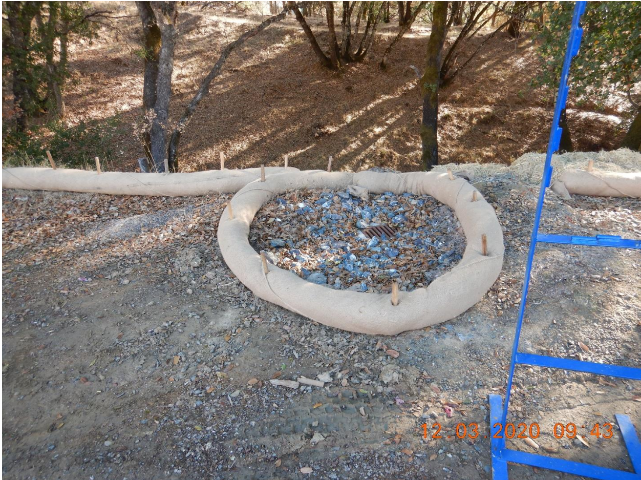
Picture 2- View of a drain inlet that is protected with fiber rolls in DA-1. The fiber rolls are kept in place with wood stakes. Picture taken by Farzad Kasmaei.
