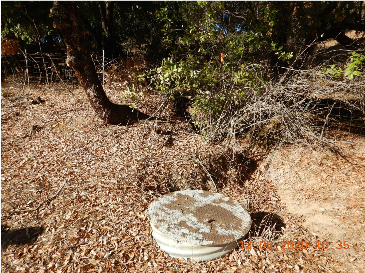
Picture 12 – View of sampling point No. 1 where the run-off from DA-1 is discharged into the shown drop inlet via the swale shown. Picture taken by Farzad Kasmaei.
