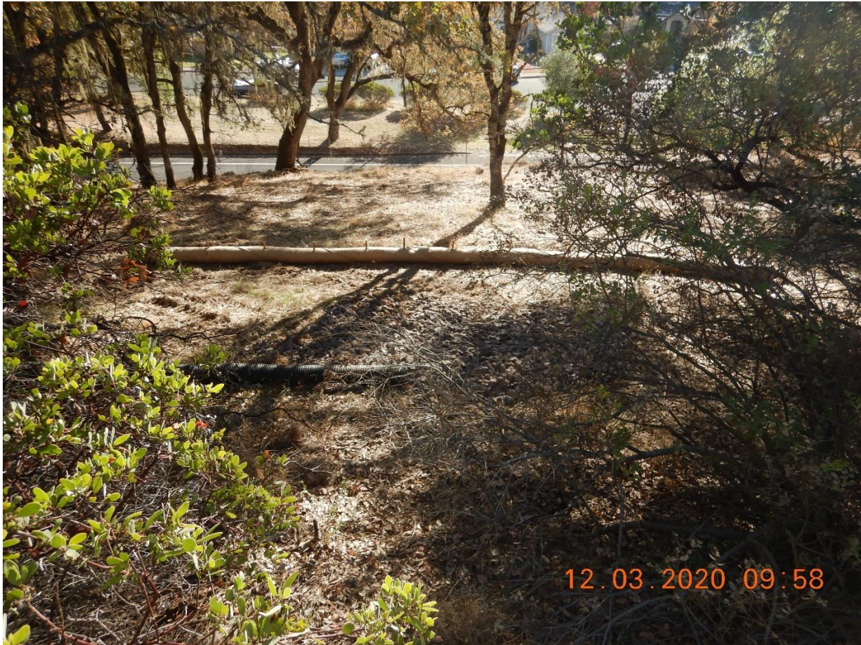
Picture 7- View of a black pipe that receives the runoff from the pistol area shown in Picture 6 and discharges the water on the rip rap area where a fiber roll has been installed down gradient of the hill side. Located in DA-2. Picture taken by Farzad Kasmaei.
