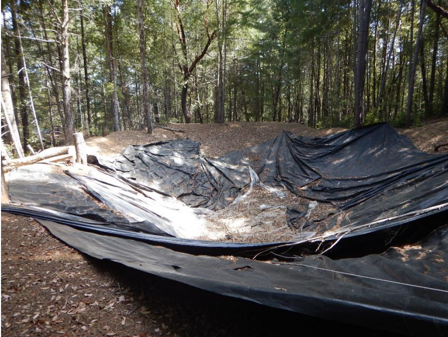
Photo 3: Dry, tarp-lined pond uphill of cultivation area
