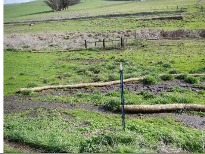
Straw wattles in pasture below and southeast of waste tank and holding pens.
