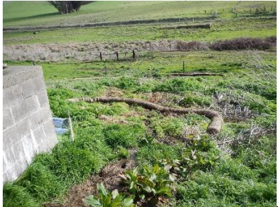
South side of waste tank with straw wattle below
