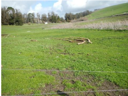
Straw wattles in pasture below and northeast of waste tank.
