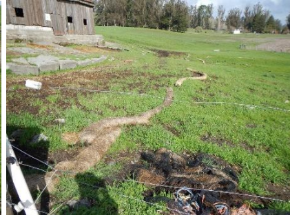
Straw wattles in pasture north of waste tank and below hay barn (left)
