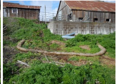
Straw wattles in pasture below hay barn
