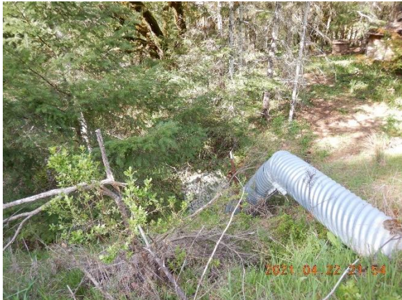
Figure 7. Pond outlet pipe downspout to channel with rock recently placed.
