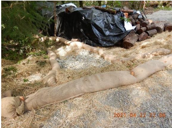
Figure 11. The outlet of the culvert with interim erosion control.
