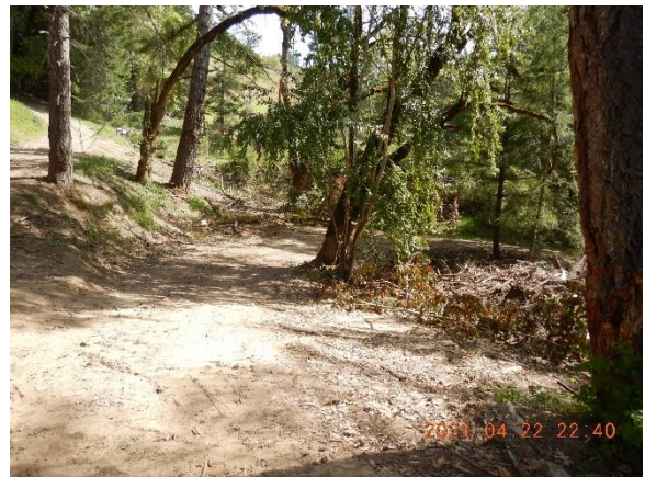
Figure 14. View of access road with pond upslope to left and slash in watercourse downslope.
