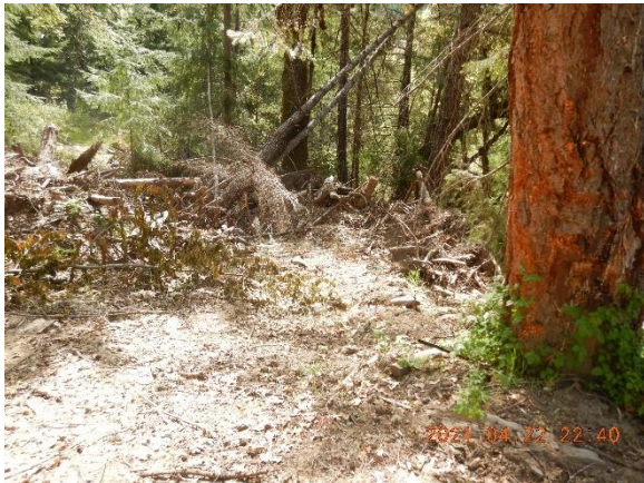
Figure 16. WQ5, slash and sediment in watercourse below road, to be cleaned up and road decommissioned.
