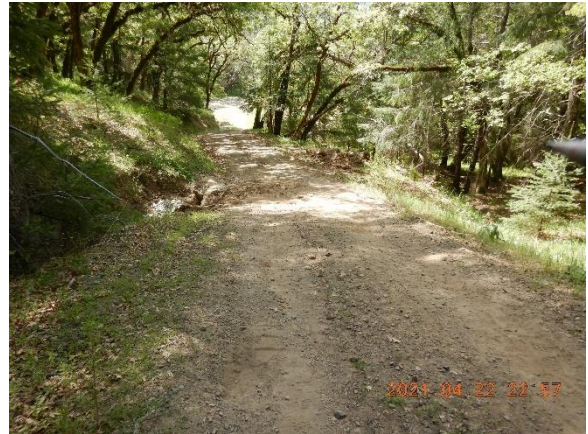
Figure 21. Crossing at WQ7. Minimal fill, low gradient watercourse below road.
