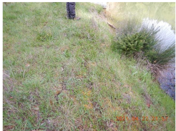
Figure 6. Cracks in berm near outlet pipe.
