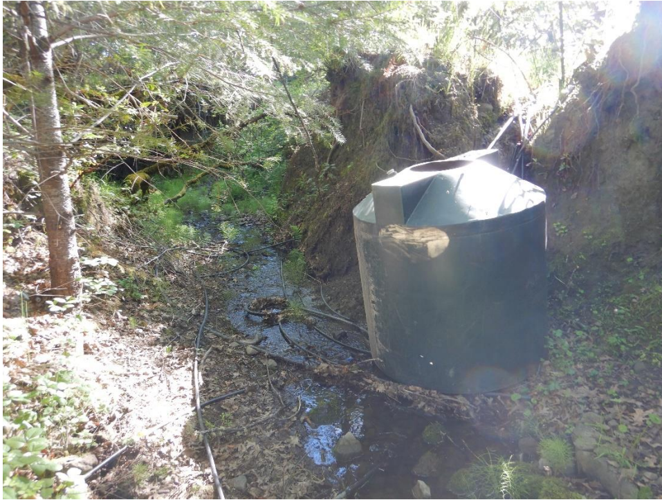
Photo 7—Water tank in the vicinity of WQ3, and pictured in previous image, is within the banks of the watercourse.
