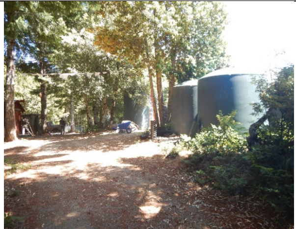
Photo 4: water storage tanks at WQ4
