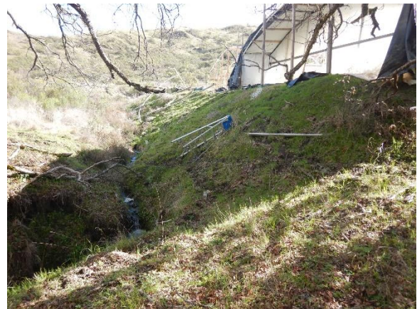
Figure 11. Cultivation flat fill face encroaches on watercourse.
