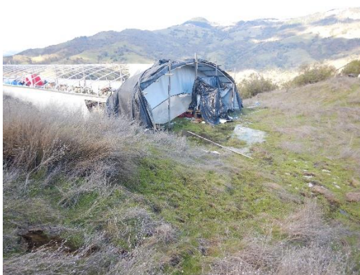
Figure 19. Greenhouse is built in flow path of watercourse.
