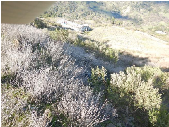
Figure 17. Looking downslope from the berm of Pond B, a greenhouse is built along the flowline of the watercourse.
