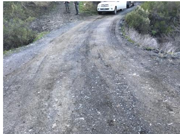
Figure 24. Convergent roads at watercourse crossing are hydrologically connected to watercourse and deliver sediment to watercourse.
