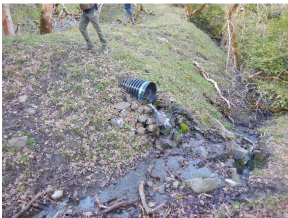
Figure 9. Pond A has an 18 inch outlet pipe through berm to watercourse (398).
