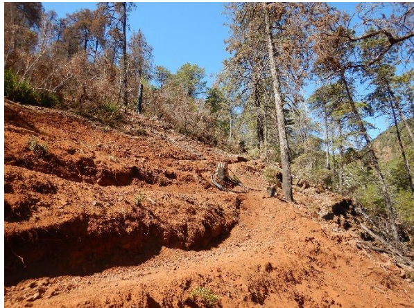
Photo 6: View of smaller terrace construction located at WQ4.
