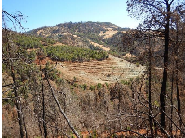
Photo 8: Wider view of the terrace construction as seen from WQ4.
