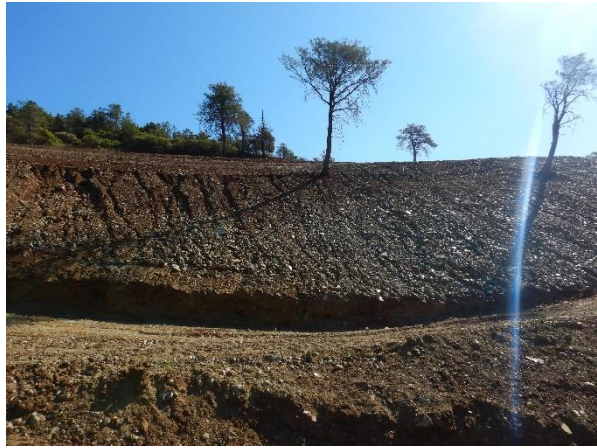
Photo 4: View of rills forming on terraced hillside at WQ2.
