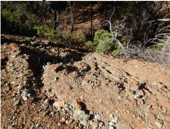
Photo 5: View of spoils and rills adjacent to terracing at WQ2.
