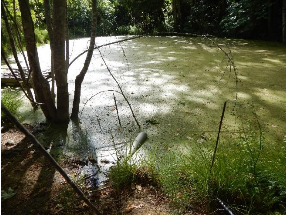
Photo 15: View of the inlet of the pond outflow pipe.
