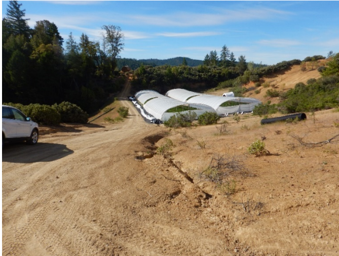
Photo 1 - Cultivation Area 1: Rut on steep dirt access road to four hoop houses
