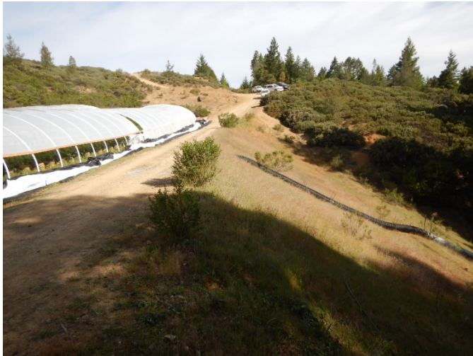
Photo 2 - Cultivation Area 1: Culvert directs irrigation and road runoff downhill
