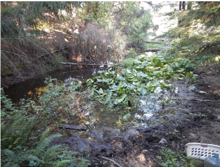
Photo 6: GG6: Onstream, unlined pond with culvert set high in berm
