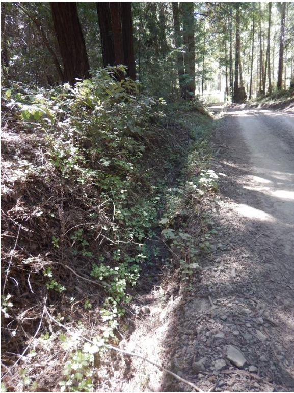
Photo 6: Diverted stream/ roadside ditch
