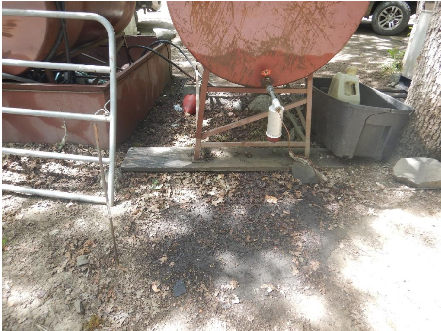
Photo 19—Diesel storage tank without secondary containment at WQ4. Patch of dark earth below the tank identifies the location of a fuel spill.
