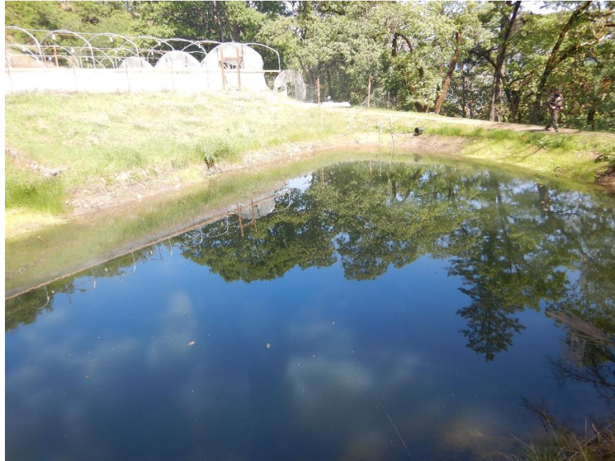
Photo 23—Looking east toward WQ 6. The reservoir outlet pipe is visible in the upper right of the image.
