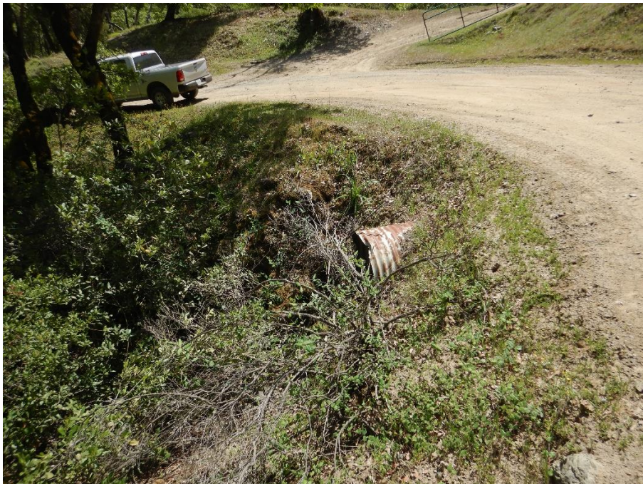
Photo 2— Looking south at 28-inch diameter culvert outlet located at WQ1.
