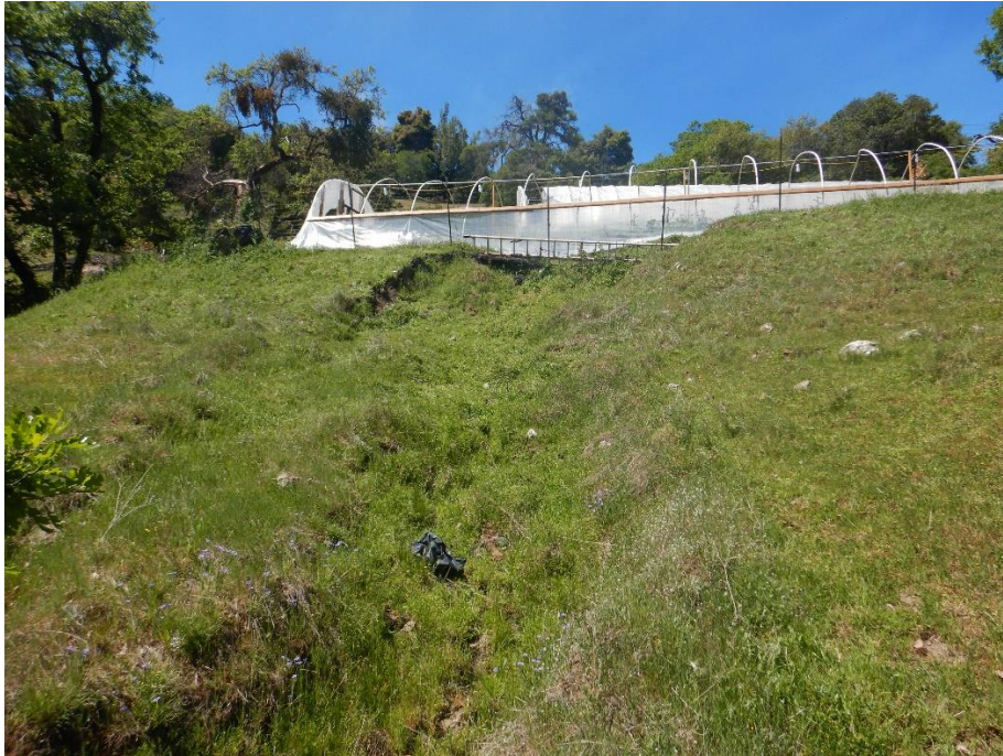
Photo 17—Looking northwest at eroded gully extending into the edge of the cultivation pad.
