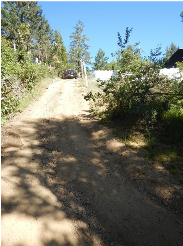
Photo 2 - Access road: Steep access road with tire ruts
