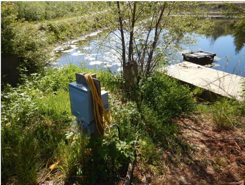
Photo 6 – Pond: Water diversion infrastructure in and adjacent to onstream pond
