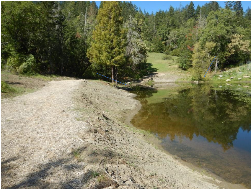
Photo 4 – Pond: Disturbed area on pond bank. The approximate locations of Class III watercourses entering the pond are marked by blue arrows
