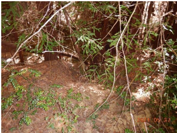
Figure 19. WQ2. Sediment deposition along flow path to watercourse.
