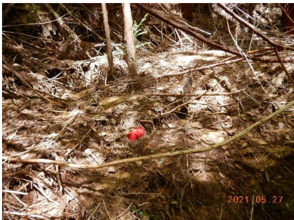
Figure 20. WQ2. Sediment deposition along flow path to watercourse.
