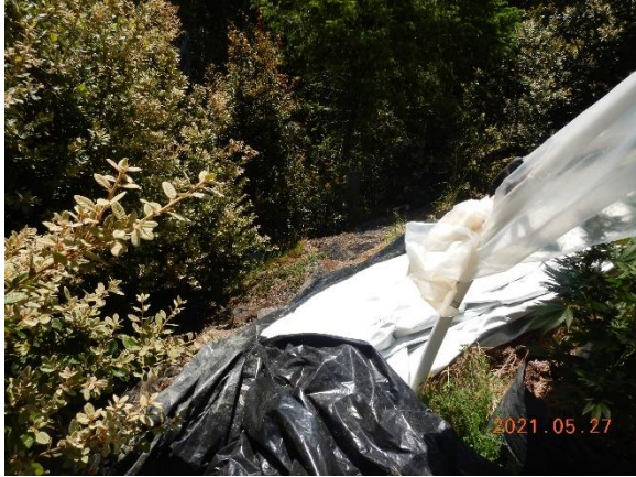
Figure 12. Oversteepened fill at CA2, WQ1.
