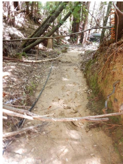
Figure 22. Channel is buried in discharged fine sediment that settled as bottom deposits. Likely much sediment transported downstream with flows.
