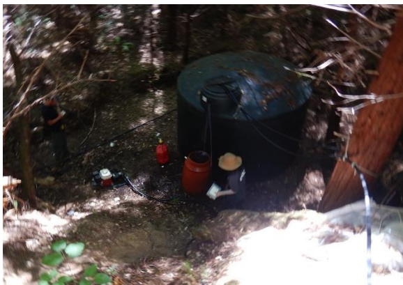
Figure 24. WQ3. Water is diverted from spring to tank, located on stream bank, with overflow running on ground, with gas pump in flowpath.
