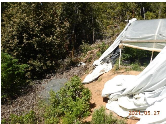
Figure 14. WQ1. Oversteepened fill at CA2 is pushed onto slash, both have eroded and slipped down slope.
