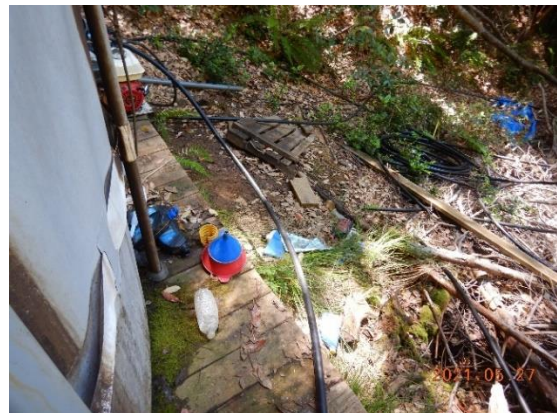
Figure 28. Oil containers and gasoline without containment in watercourse
