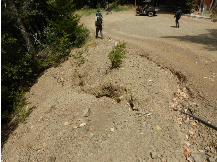
Photo 7: LL5: Surface erosion on steep portion of access road
