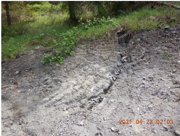
Figure 5. Cut bank of fresh graded area near 489.
