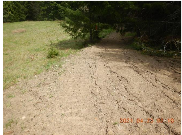
Figure 8. New road construction between 489 and 490.
