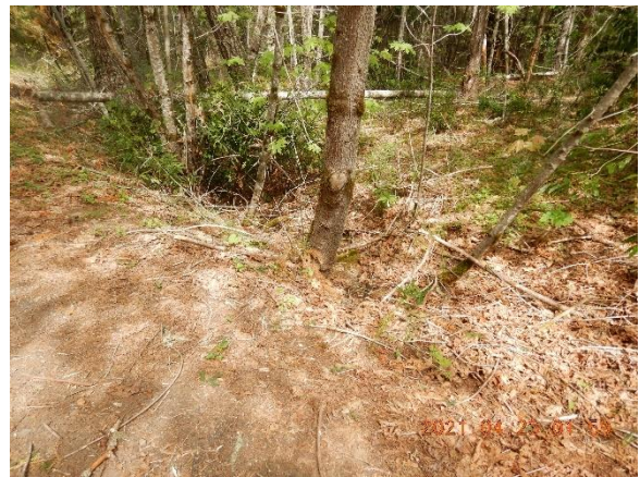
Figure 3. 488- Class III road crossing culvert outlet.
