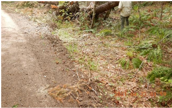
Figure 2. 488- Class III road crossing culvert inlet.
