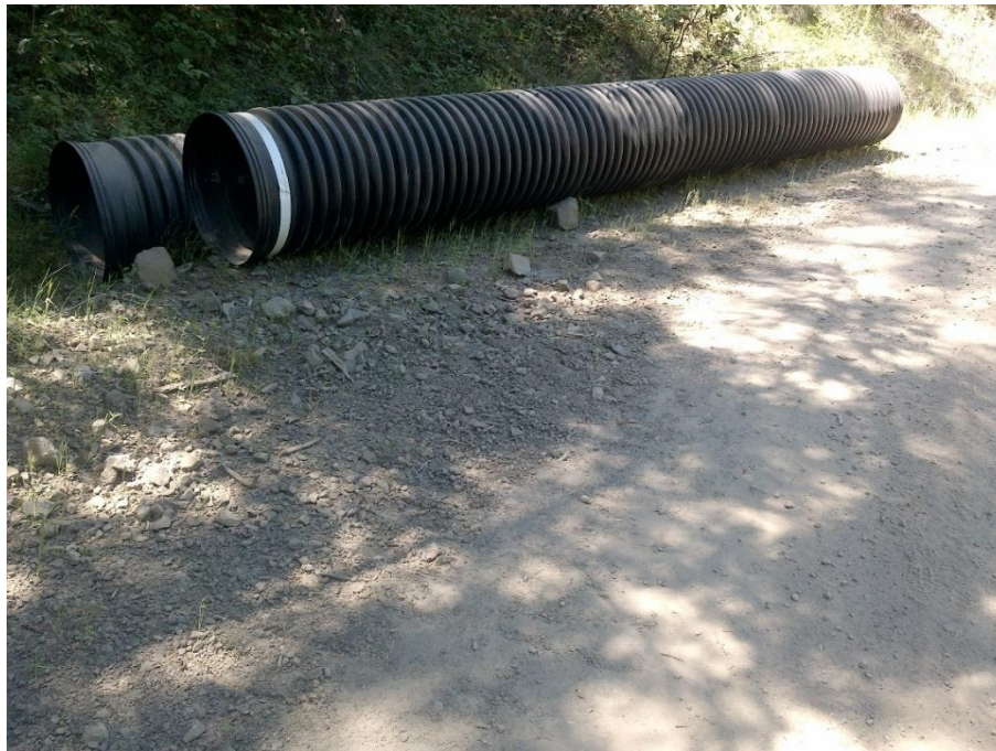
Photo 14— Two new 28-inch diameter pipes staged near WQ7.
