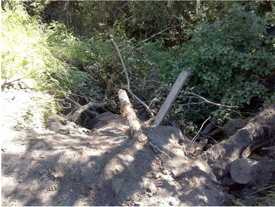
Photo 3—Earth and woody debris pushed into watercourse at WQ2
