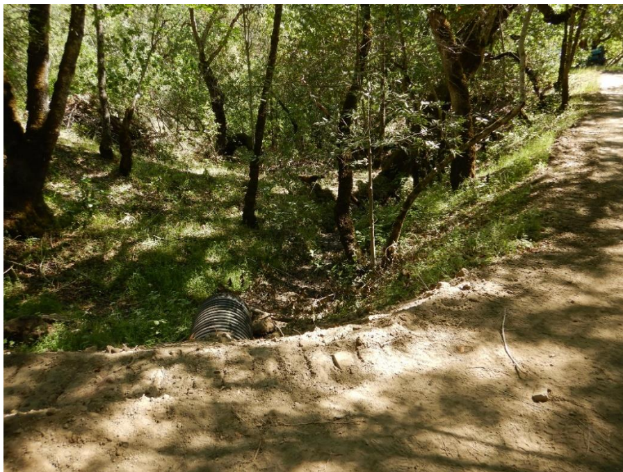
Photo 2—Looking west and downstream at recently installed culvert at WQ1.
