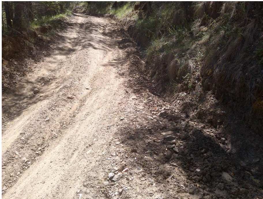
Photo 10— Steep rutted road at WQ5. A roadside trench in the middle of the image is directed to the watercourse in the following image.
