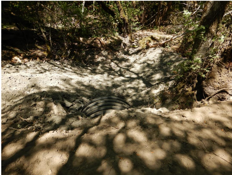
Photo 7— Looking upstream at recently installed 60-inch diameter culvert at WQ2.
