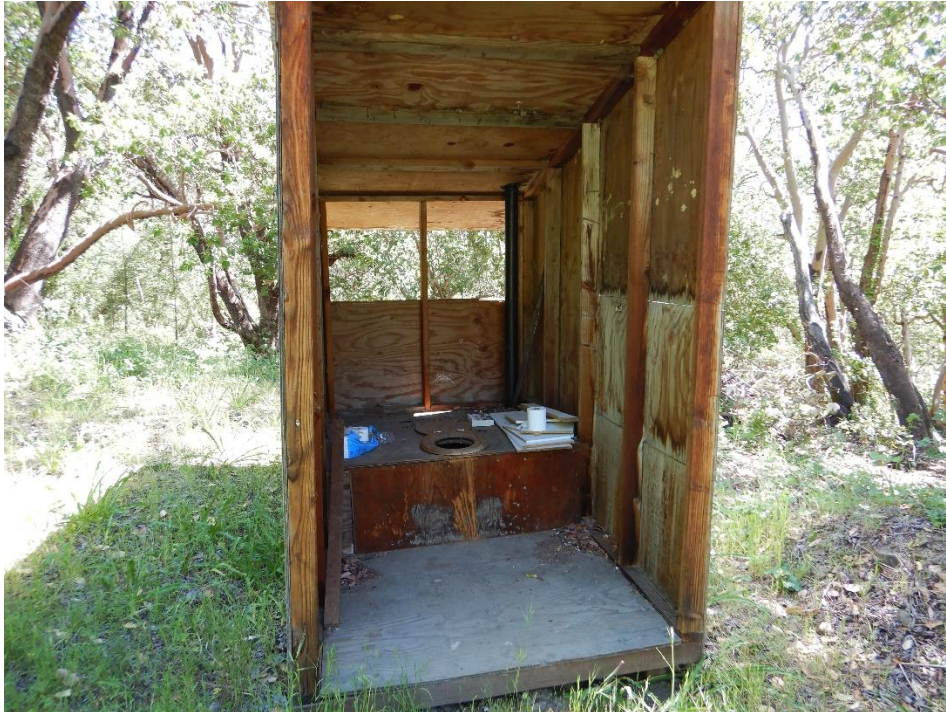
Photo 8—Pit toilet at located at WQ3.
