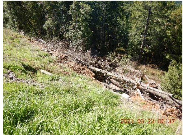
Figure 9. Upper graded flat, near GPS Point 447, slash at toe of fill slope.
