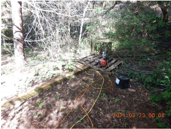
Figure 7. Water pump connected to waterlines running through culvert at GPS point 445.
