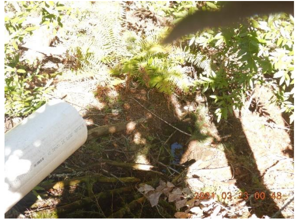
Figure 13. GPS location 449. Trench in previous figure outlets to a pipe that discharges over slope above pond; trench and pipe have potential to carry pollutants to the pond, which provides aquatic habitat and discharges to surface waters.
