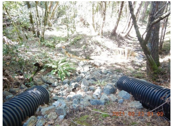
Figure 18. At base of pond berm, outlet pipes drain to watercourse. The LSA included the rock placement.
