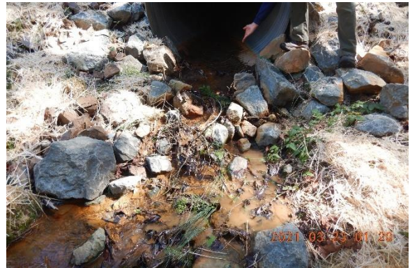
Figure 21. GPS location 455. Outlet of Crossing 3 with evidence of sediment deposits in downstream channel. According to CDFW, the erosion control measures weren't installed at the time of there inspection in December 2020.
