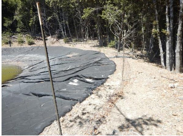
Photo 2: View of the pond outflow infrastructure.
