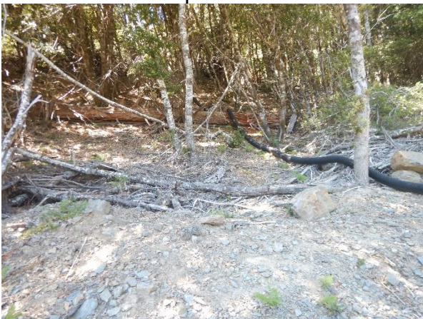
Photo 5: View of pipe coming down the hillside above the pond.
