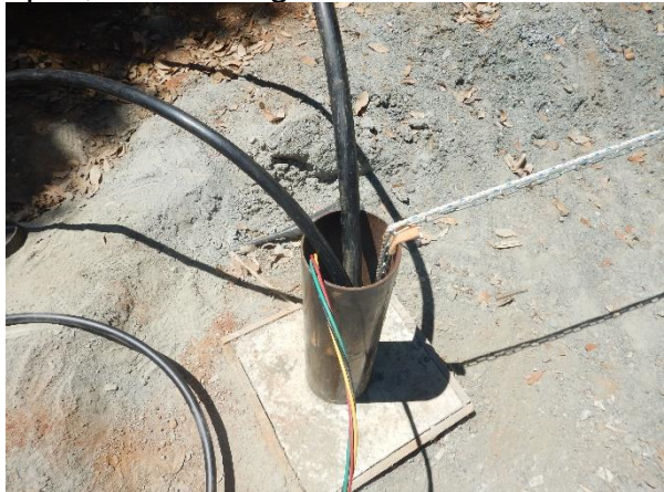
Photo by Ermias Berhe, NCRWQCB Photo 18: Closer view of the open, uncovered groundwater well.
