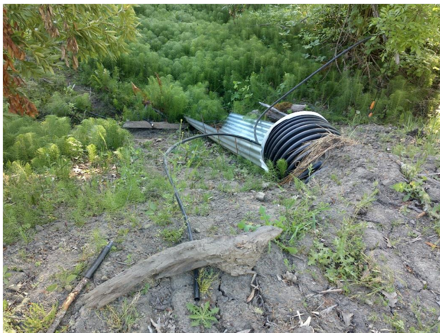
Photo 4—Reservoir outlet pipe, at WQ1, directed onto a corrugated metal trough on the impounding buttresses' outboard face. Plant genus Equisetum is growing in a dense patch at the bottom of the trough.
