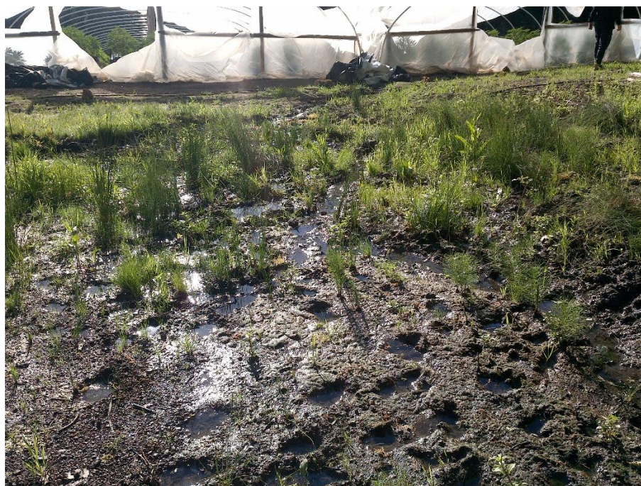
Photo 17— Looking south from the same location as the previous image. Water leaking from the reservoir has saturated the ground and flows into greenhouses in the background of the image. Plant genera Juncus and Equisetum are growing in the saturated ground.
