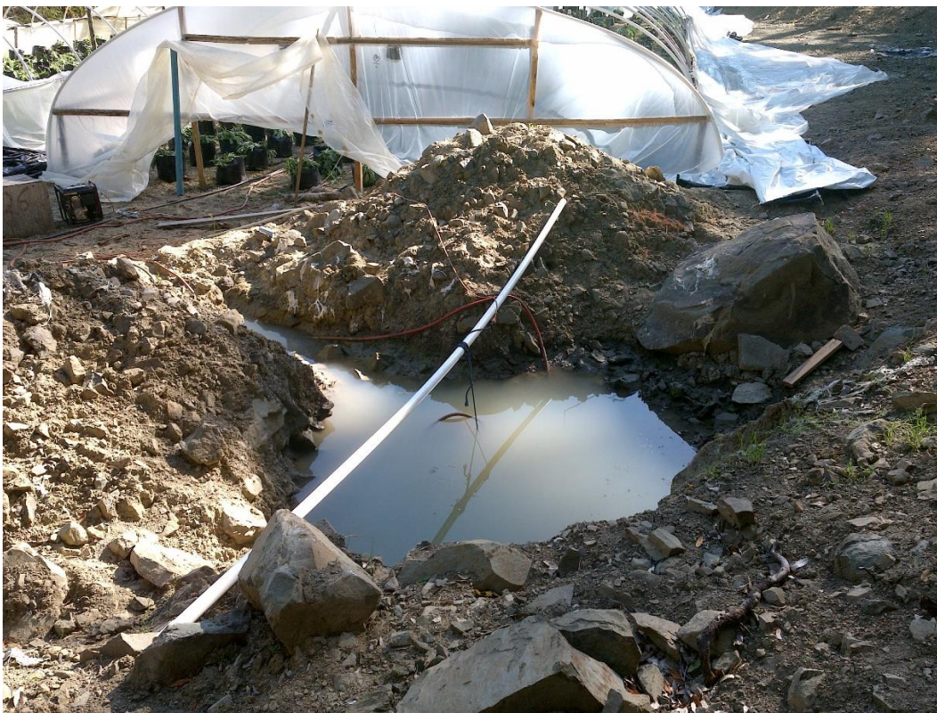
Photo 26—Pooled water in an excavated hole on the western edge of the cultivation pad at WQ8.
