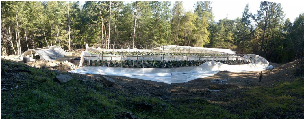
Photo 25—Looking north at recently constructed cultivation pad at WQ8.
