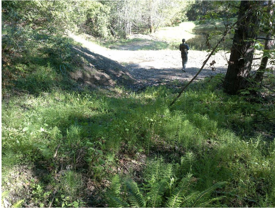
Photo 13— Looking downstream where drainage from previous image intersects the southwestern berm of the reservoir.
