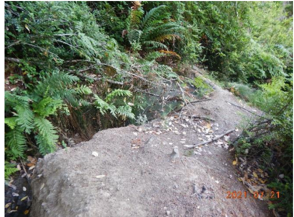
Figure 6. Excavation of spring at WQ1 with bermed outlet.
