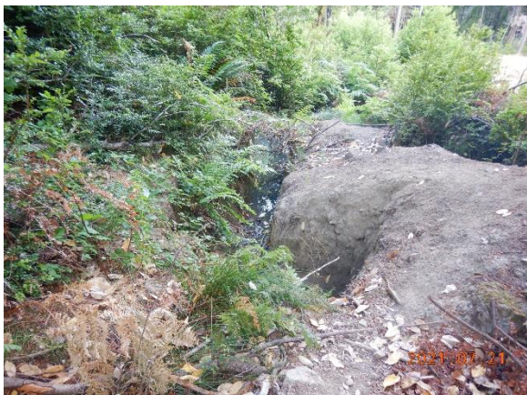
Figure 5. Excavation of spring at WQ1.
