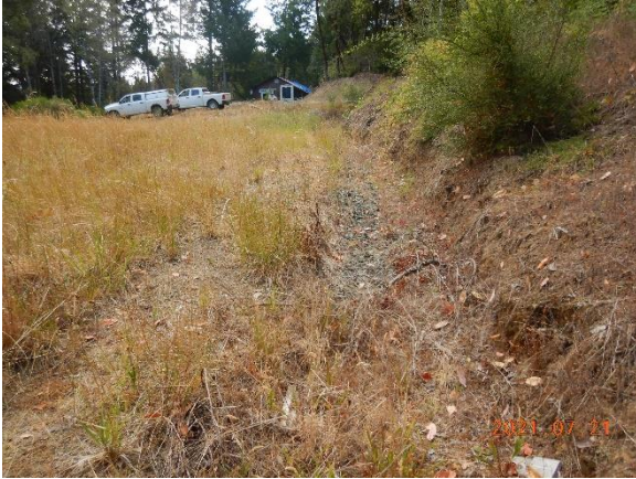
Figure 9. The edge of the flat has what appears to be a French drain capturing flow.
