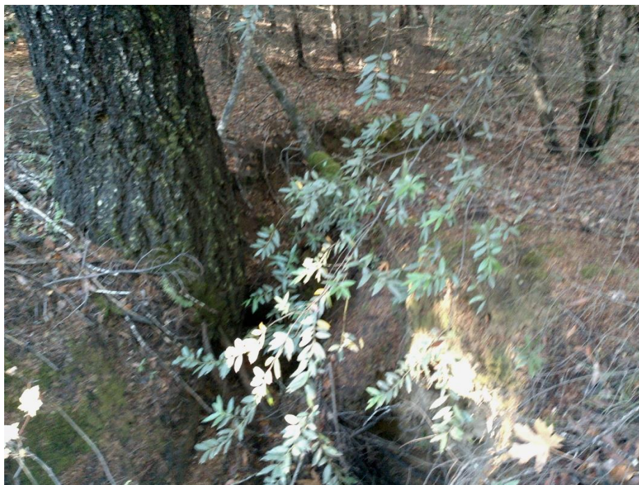
Photo 15—The watercourse downstream from culvert pictured in previous image at WQ 10.
