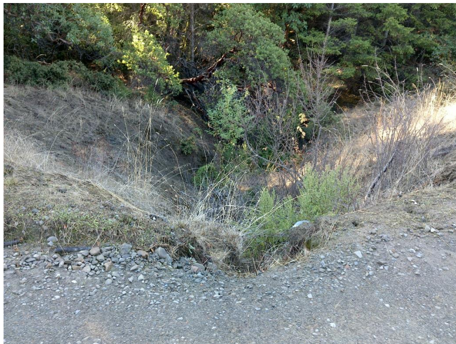
Photo 4—Looking south and downhill at culvert outlet located at WQ 3.
