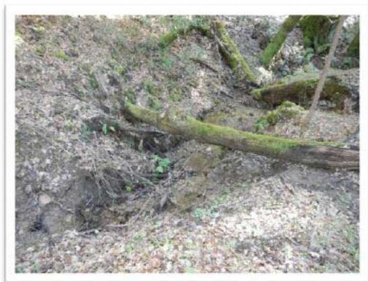
Culvert C4 inlet and channel below outlet (photos taken by DFW)
