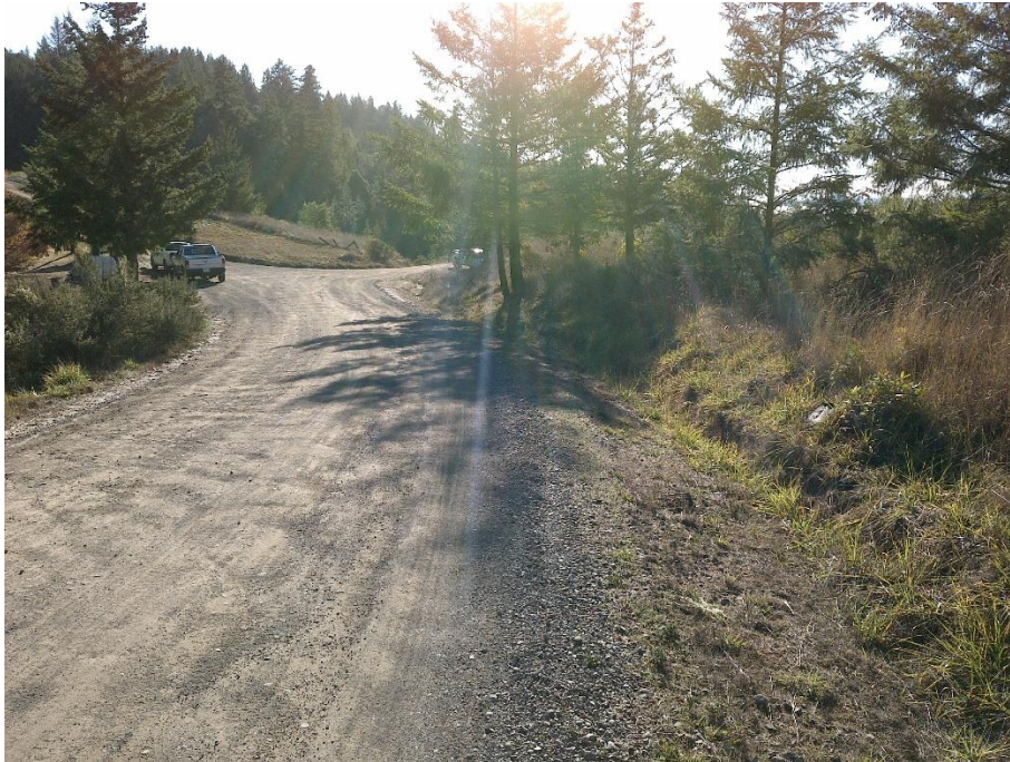
Photo 1—Looking south from WQ 1 toward WQ 2. Road collects stormwater and discharges to inboard ditch, shown in the right of the image before discharging into incising channel at WQ 2 pictured in the below photo.
