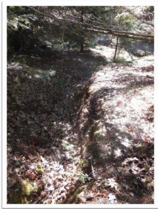
Gully, looking south
