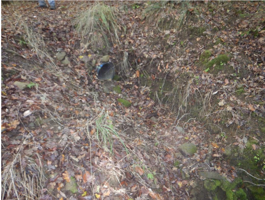
Photo 35—Looking north at culvert outlet in the vicinity of WQ 21. The culvert is aligned with the stream bottom.
