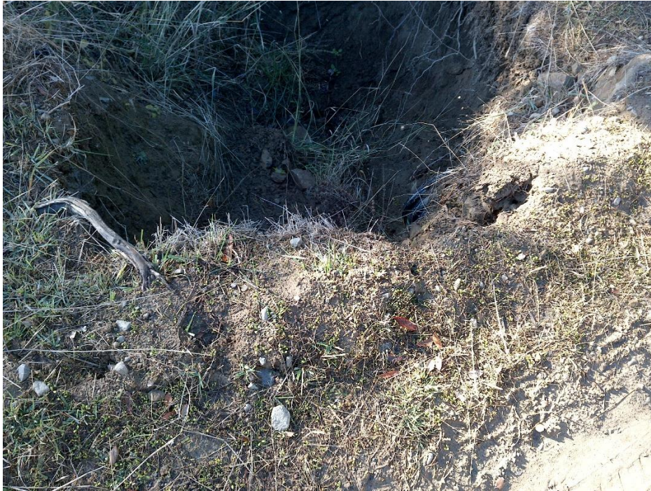
Photo 7—Looking south at culvert outlet at WQ 5. The top of the culvert is visible to the center-right of the image.
