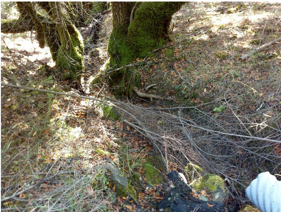
Photo 8—Looking west at culvert outlet at WQ 6.
