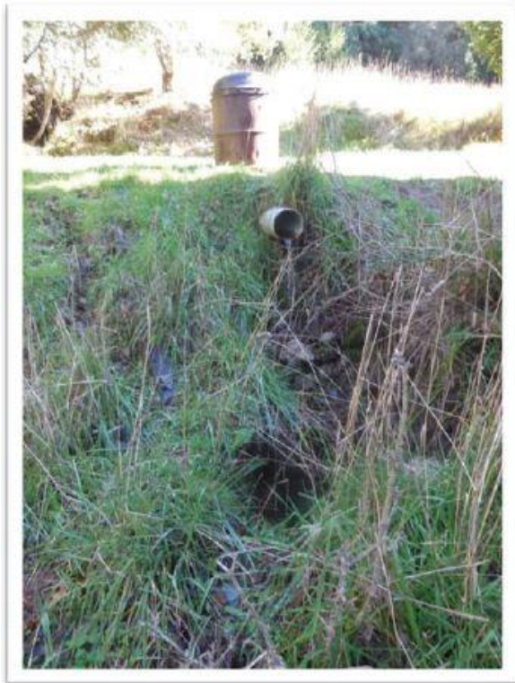
Culvert C1 – outlet and eroding channel below
