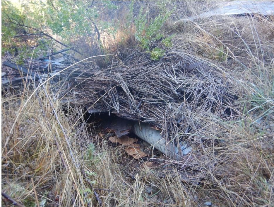
Photo 21—A buried culvert where a legacy road crosses the watercourse at WQ 13.
