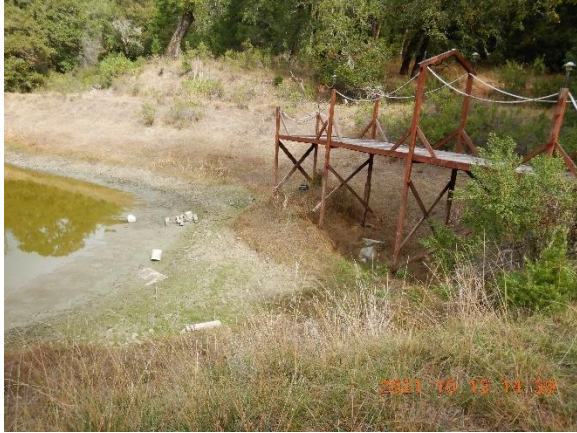
Figure 15. Dock located in Pond 1.
