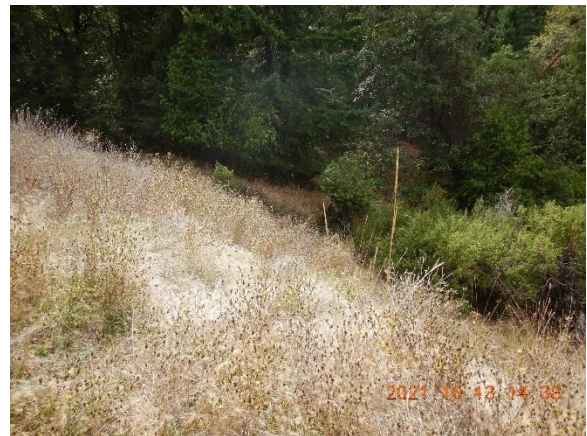
Figure 13. The exterior slope of earthen berm associated with Pond 1 is vegetated.
