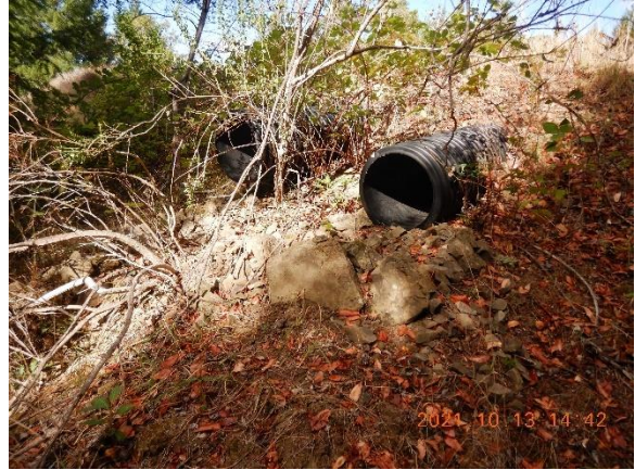
Figure 18. Outlets of Pond 1 discharge pipes onto hillslope.
