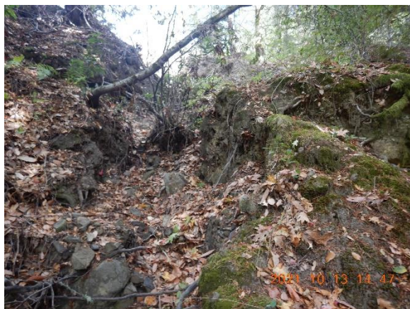
Figure 21. Lower portion of gully associated with pond overflow pipes.
