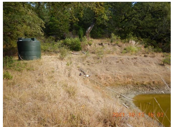
Figure 14. Picture of a gas pump for water transfer from pond to tank.
