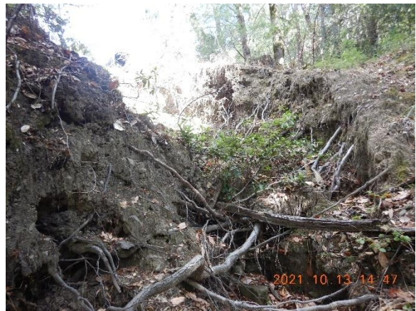
Figure 20. Active middle portion of gully associated with pond overflow pipes.
