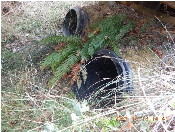
Figure 16. Pond side of two parallel 24" outlet pipes, located high on slope.
