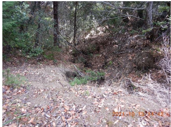
Figure 19. Tio of gully formed at outlet pipes.
