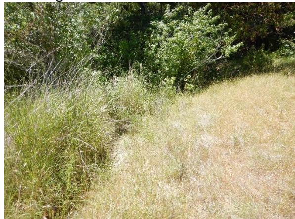
Photo 10: View of hillside drain that discharges to a Class II watercourse.
