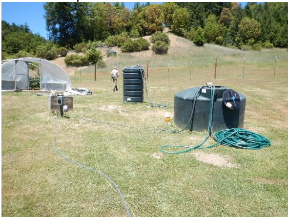
Photo 9: View of water storage tanks near the top of CA1.
