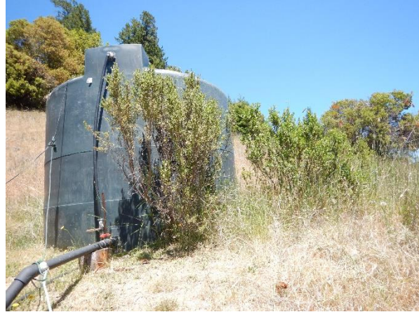
Photo 8: View of adjacent water storage tank located on the hill above CA1.
