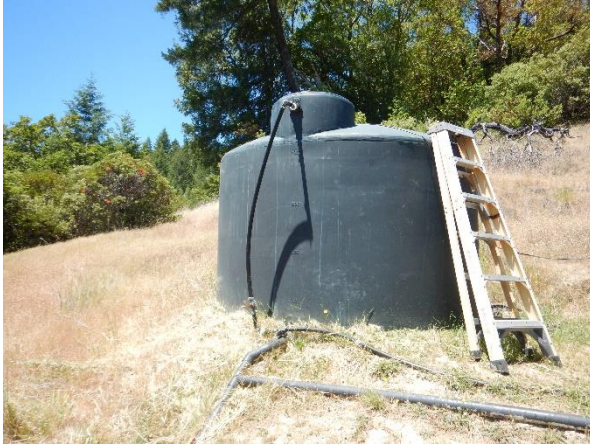
Photo 7: View of water storage tank located on the hill above CA1.
