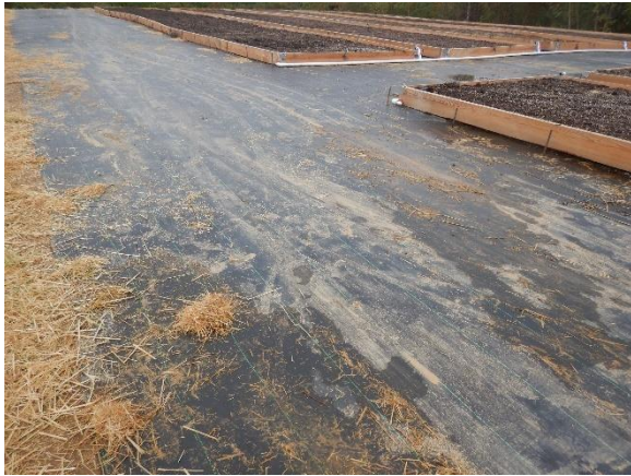
Figure 8. Woven plastic fabric likely holds water which, then drained to initiation point.
