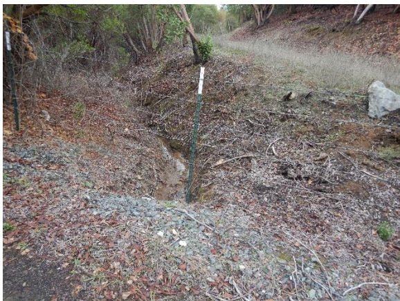
Figure 29. The Class III watercourse and road are parallel and at the base of the driveway, the watercourse enters a functional culvert.
